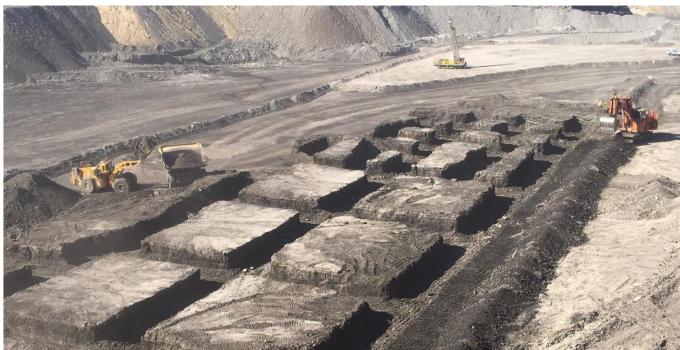
Figure 5-2: Cleaning of waste material between coal pillars (New Hope Group, 2021)
