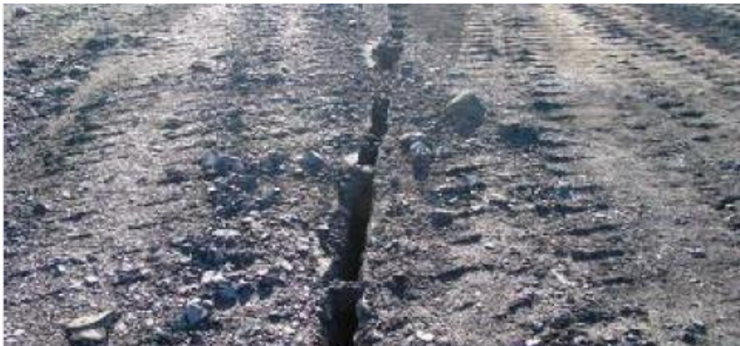
Figure 2-13: Open crack on the burden above underground workings (Miller, 2008)
