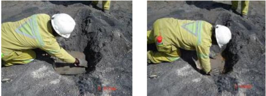
Figure 2-17: Sealing of over-drilled holes with a steel plates (Nel, 2008).
