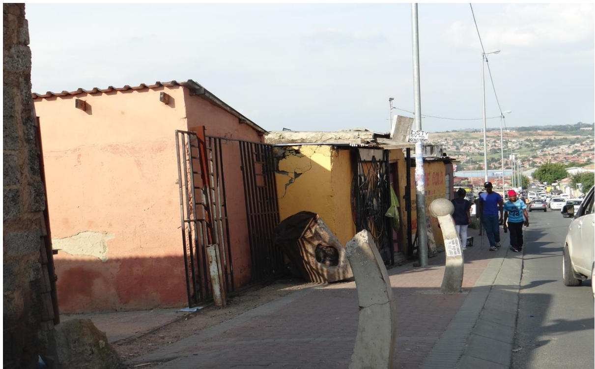
Annexure Picture 6: Structures built in contravention of building line restrictions (Ismail, 2017)
