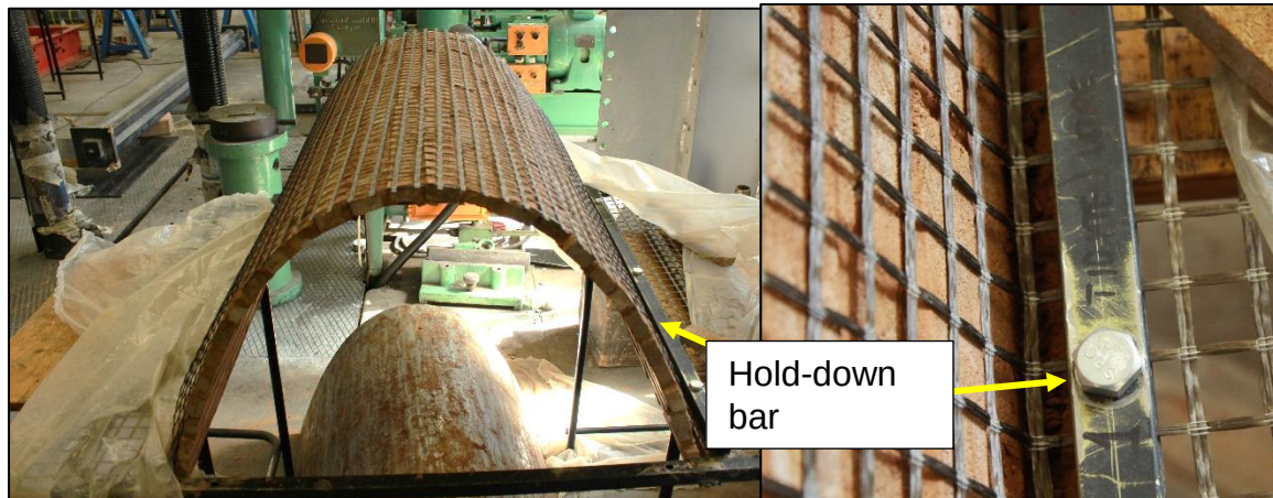
Figure 5.21: Geogrid laid over the arch and secured on either end
