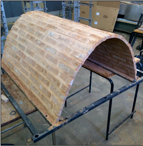
Figure 4.23: Arch cured and transverse bearer bars installed
