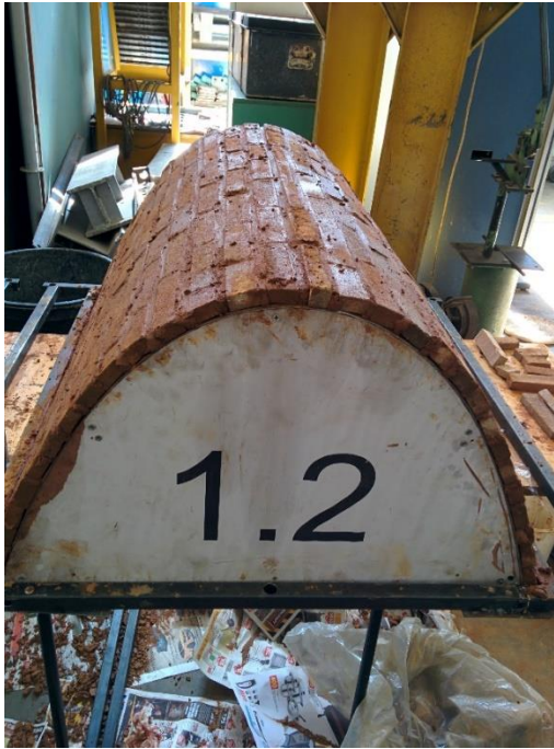
Figure 4.21: Arch built over formwork
