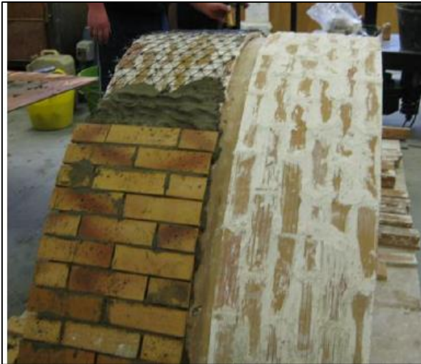
Figure 2.22: Reinforced and unreinforced arches during construction (Terry, 2011)
