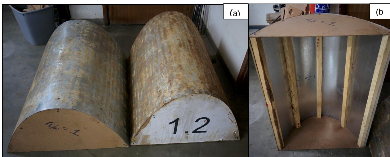
Figure 4.7: Formwork used for the construction of the arches: (a) top of formwork (b) underside of formwork
