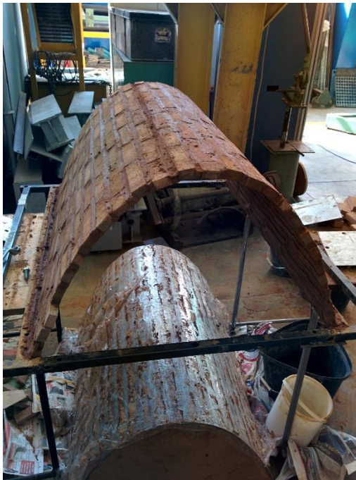
Figure 4.22: Formwork removed from arch
