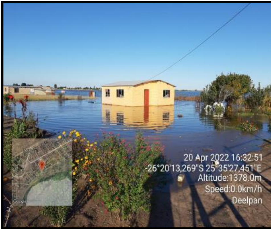
Figure 4.3: Over flooded RDP houses in the Deelpan Village. Images captured in April 2022 of RDP structures affected by the floods Source: Community representative member.
