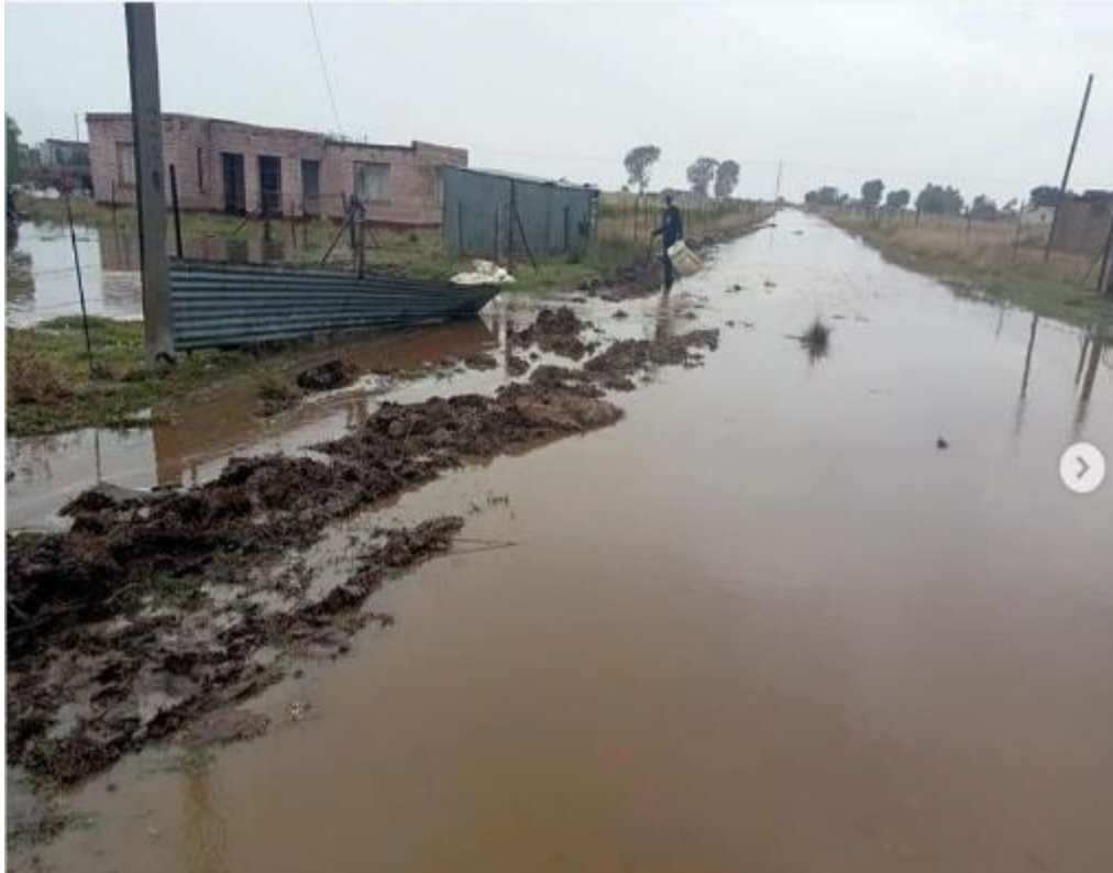
Figure 4.4: Over flooded roads in the Deelpan Village. Images captured in April 2022 during the flooding days. Source: Community representative member.
