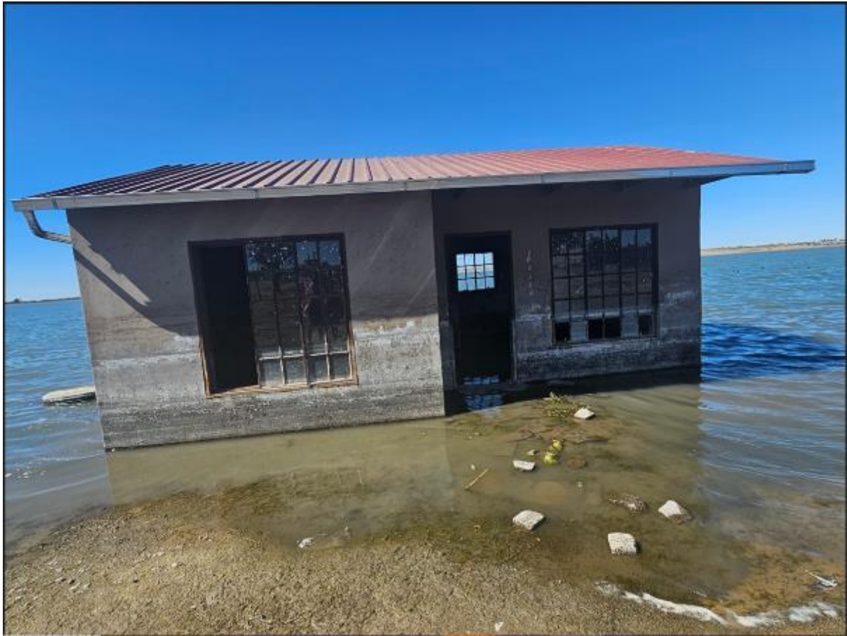
Figure 4.7: Over flooded house in the Deelpan Village. An image captured on the 23rd of September 2023 after the flooding. Source: Author.
