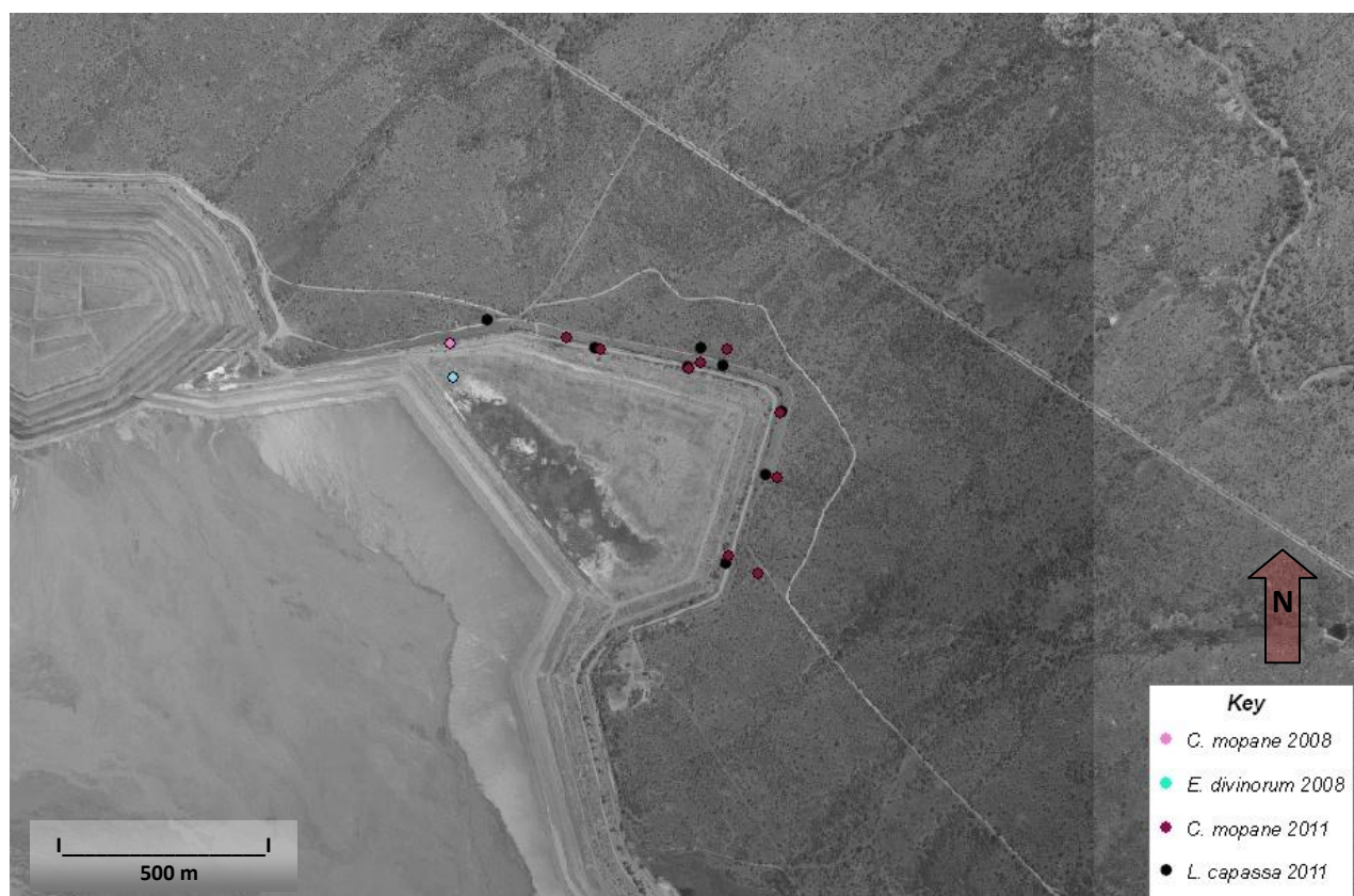
Figure 12: Aerial photograph showing sampling locations in the seepage area around the main Cu tailings at the Rio Tinto Palabora Mining Company (Source: Weiersbye et al. 2008)
