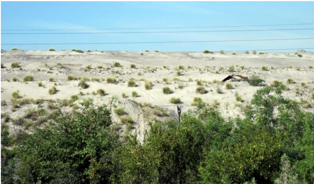
Figure 5: Side of main Cu tailings dam, Rio Tinto Palabora Mining Company
