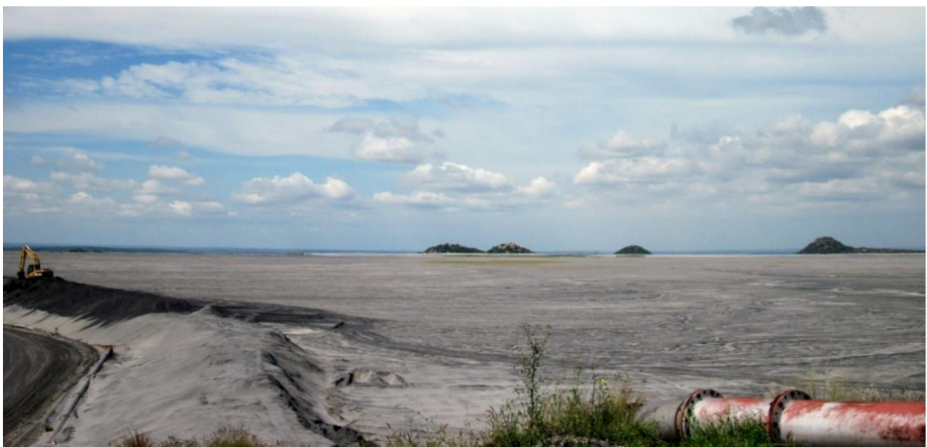
Figure 6: Top of main Cu tailings dam, Rio Tinto Palabora Mining Company
