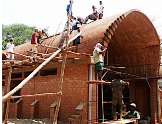
Figure 5.9 – Semi-circular vault at the Auroville Earth Institute, India
