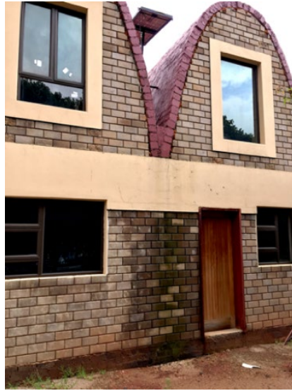
(a) East-facing wall: Outside
