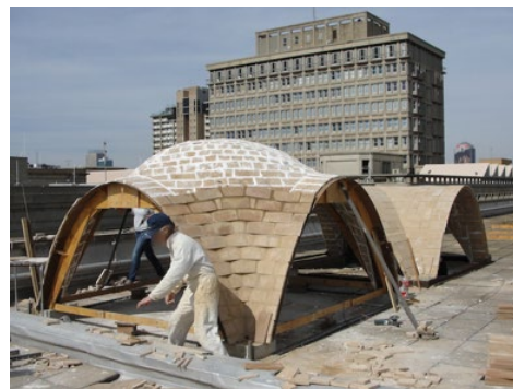
(d) Partially completed domed vault
