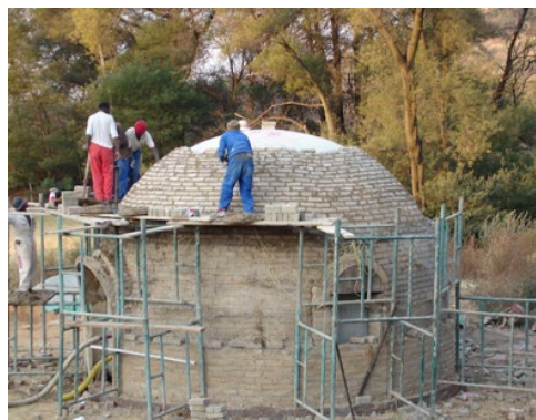
(a) Construction nearing completion
