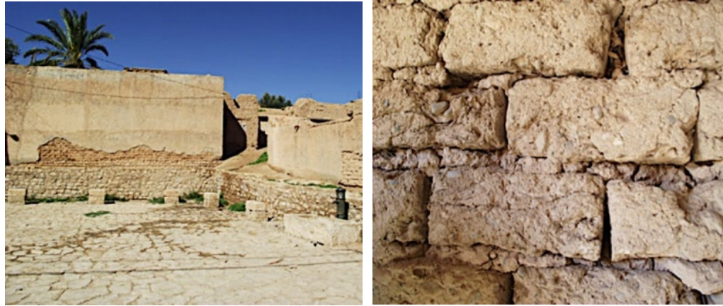
(a) Earth brick wall
