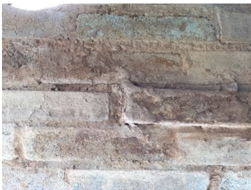
(c) Apex crack (external)
