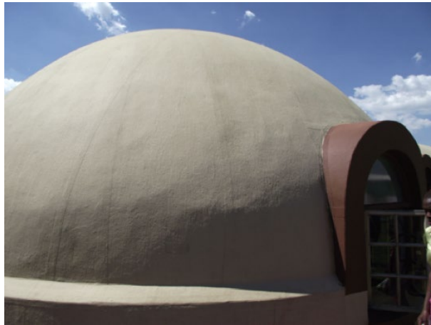
Figure 6.25 – Waterproofing membrane over a hemispherical dome
