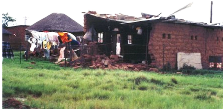
Figure 5.25 – Collapse of unsupported adobe wall of informal house (Bethany-Drakensberg, Dec. 1997) (image courtesy of Adam Goliger)
