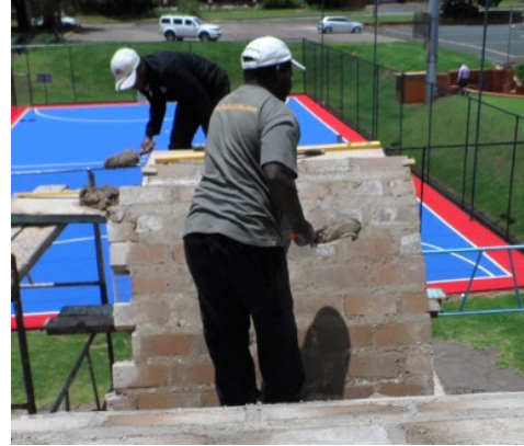
(b) Earth brick vault
