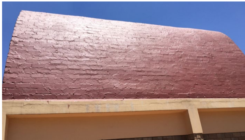
Figure 3.21 – Repaired steep catenary shells at Wits (June 2015)
