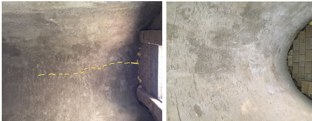
(a) Wall built up against the shell
