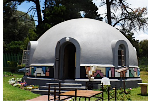
(b) Repainted dome (January, 2016)
