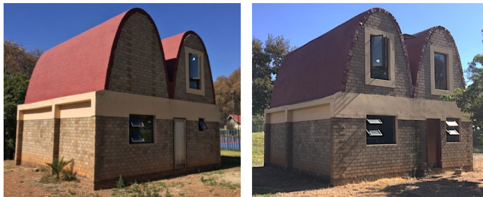
(a) Structure from the north-west
