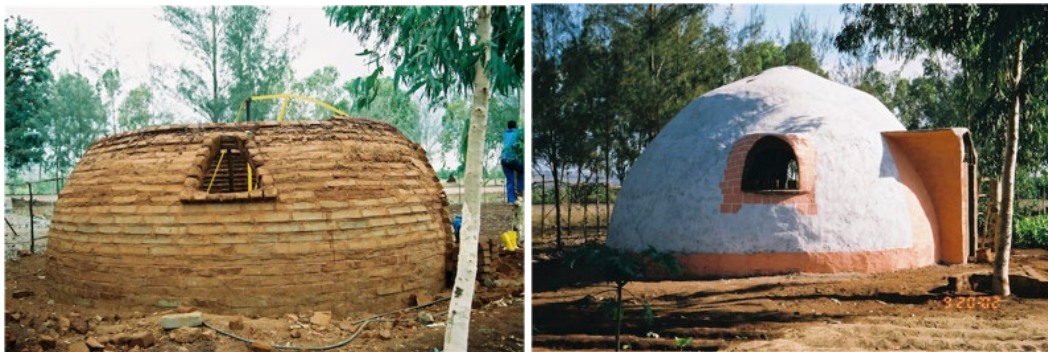
(a) Construction with cupola tracer
