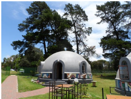
(a) CMU masonry dome
