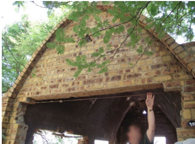
Figure 3.10 – Lintels removed from a vault in Bapong
