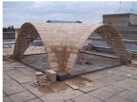
(b) Completed cross-vault
