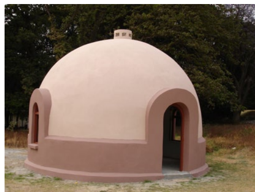
(b) Completed structure
