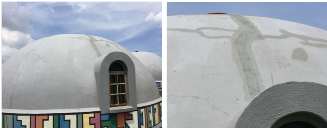
Figure 3.24 – Repairs to structural cracks in a CMU dome
