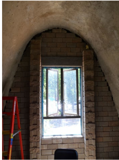
(a) west-facing wall
