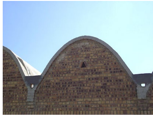
(d) Fired clay brick vaults (Bapong)
