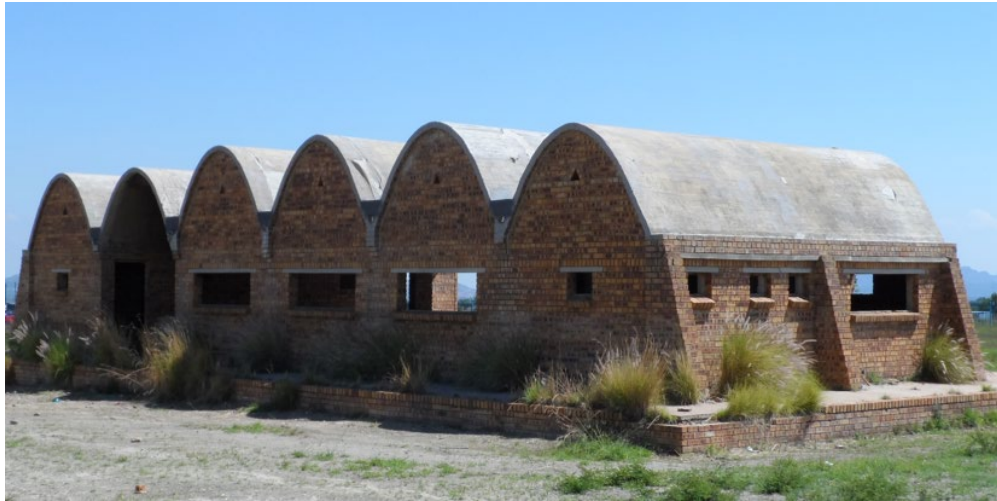
Figure 6.24 – Juxtaposition of vaults at Bapong, South Africa
