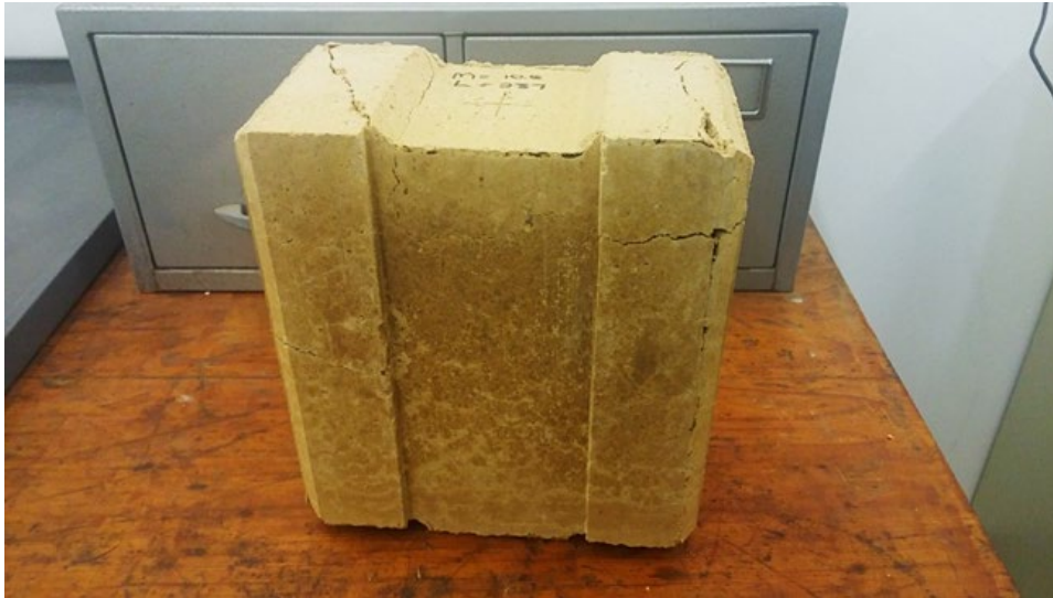
Figure 7.9 – Typical shrinkage cracking in a CSEB
