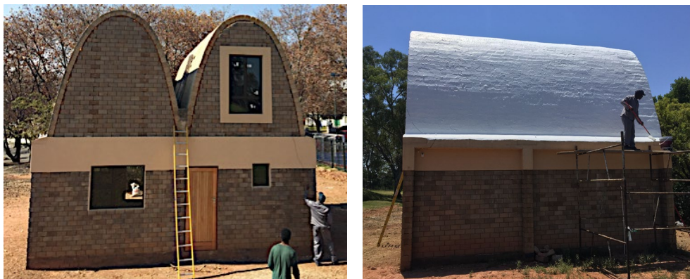
Figure 5.7 – Access onto steep catenary vaults at Wits
