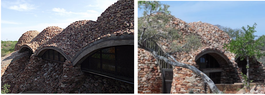
(a) Window frames fixed against the earthen shells
