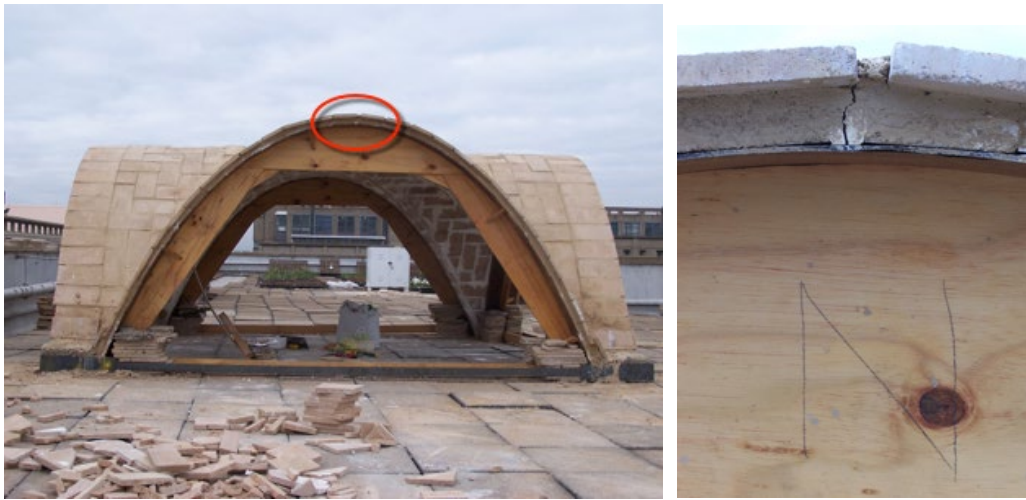
(a) Edge formwork left in place
