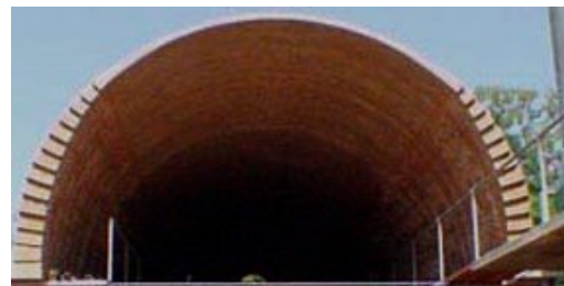
(b) Building structure
