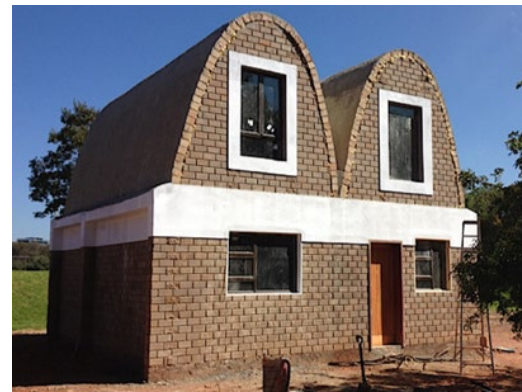
(b) Completed structure
