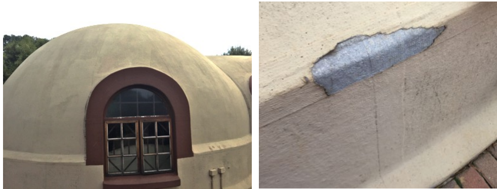
(a) Dome in good condition
