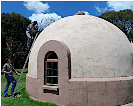
(a) Access onto a dome
