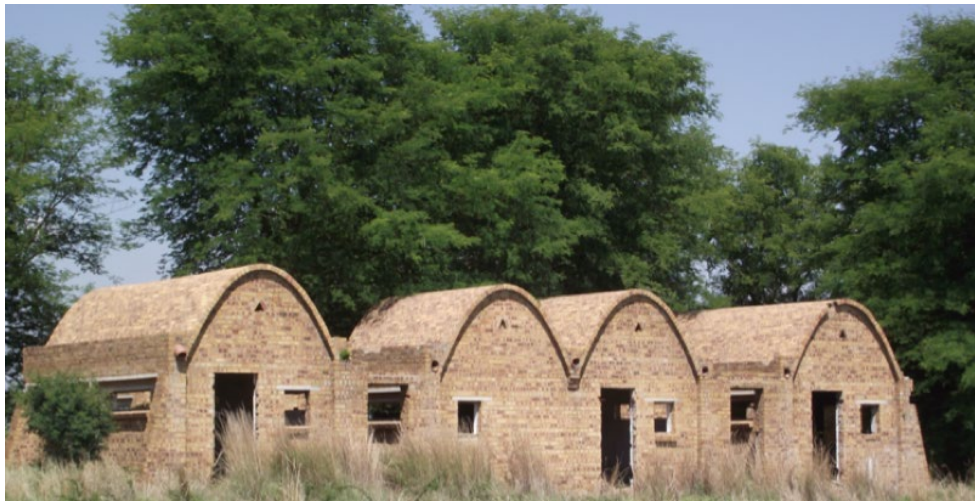
Figure 2.11 – Large trees adjacent to several abandoned vaults in Bapong, North-West
