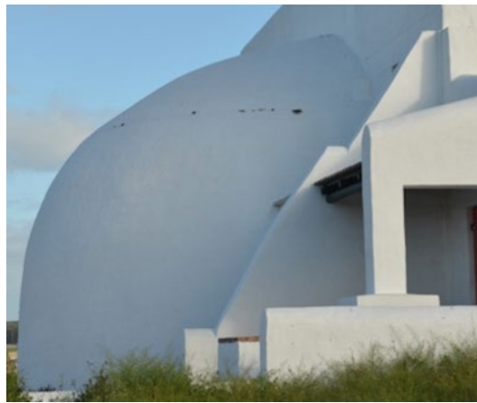
(c) Masonry half-dome: Paternoster
