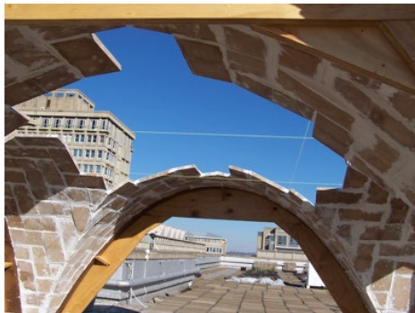
(a) Freehand construction (cross-vault)
