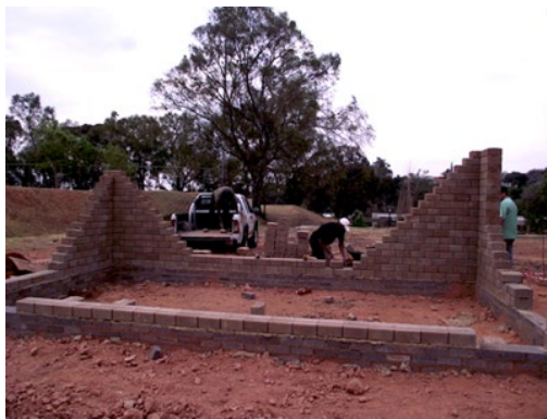
(a) Dry-stack blocks built above DPC
