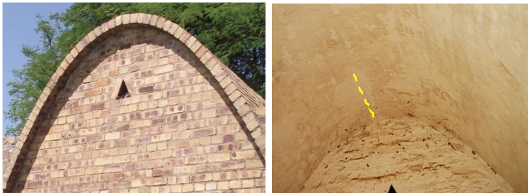
(a) Solid wall-shell connection
