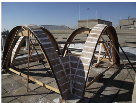
(c) Freehand construction (domed vault)
