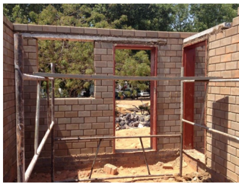
(c) Dry-stack walls
