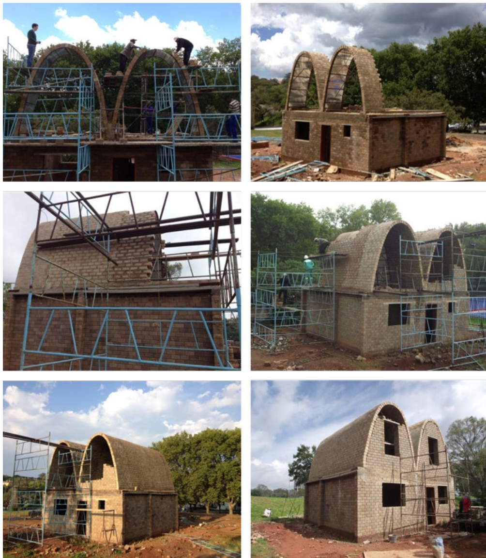
Figure 7.7 – Construction sequence of the Wits catenary vaults (images courtesy of Ivanka Bulovic)
