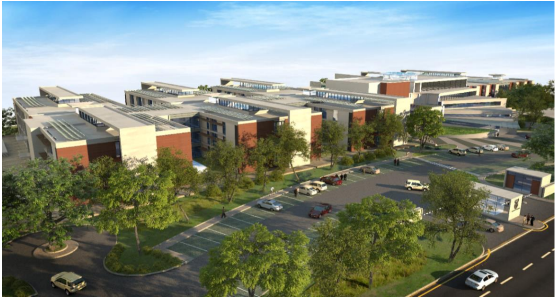
Figure 13: The DEA Building in Pretoria, Source: (DEA, 2017: 1)
