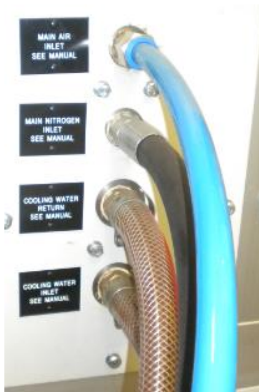
Figure 19: Supply connections
