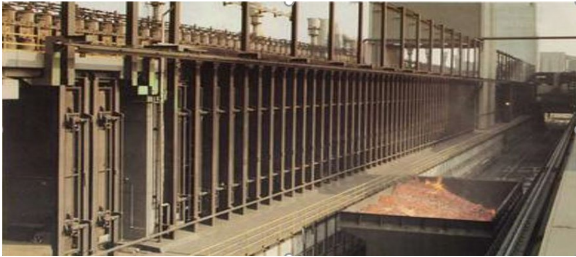
Figure 2.26: Coke Oven Operation: An oven has just been pushed and a quench car, full of incandescent coke, is en route to the Quench Station. (Photograph by Morrise, 2005).
