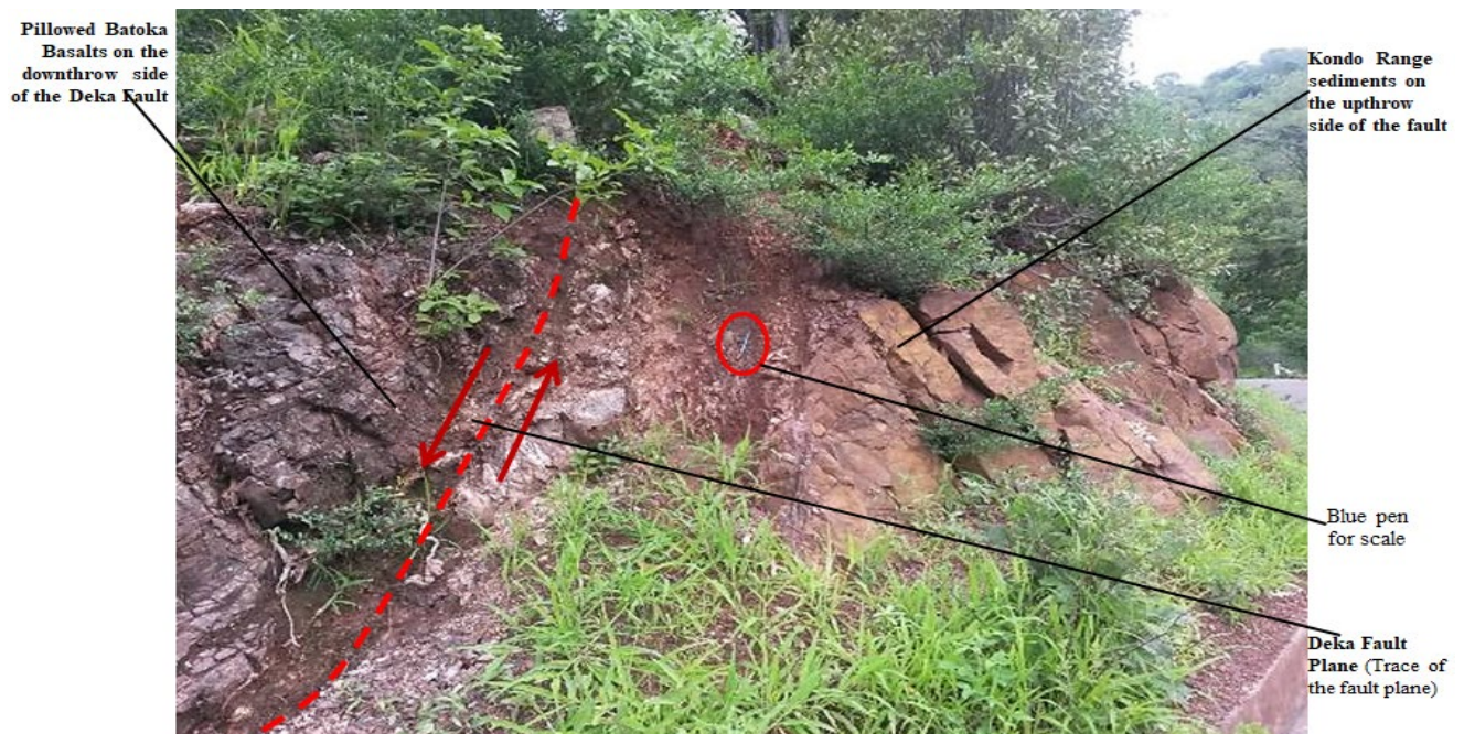
Figure 4.6: Deka Fault juxtaposing pillow lavas of Batoka Basalts (on the left) against the Escapement Grits (on the right). Location: Deka Bridge to Angling Boating Club Camp at the Zambezi River. (blue pen is included for scale).
