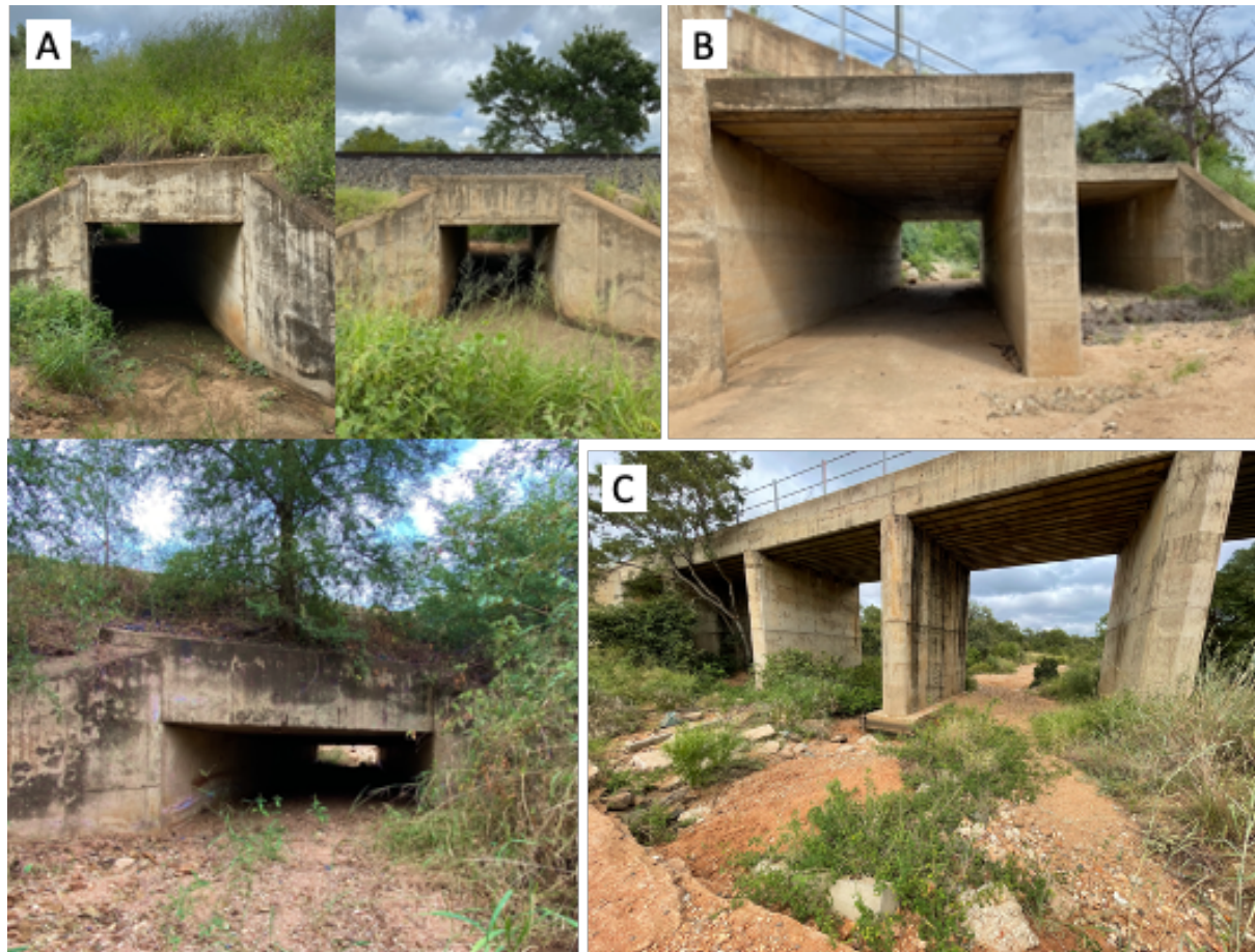
Figure 3: Examples of underpass structures in study area, in Balule Nature Reserve, South Africa: [A] box culverts [B] double box culvert [C] viaduct.
