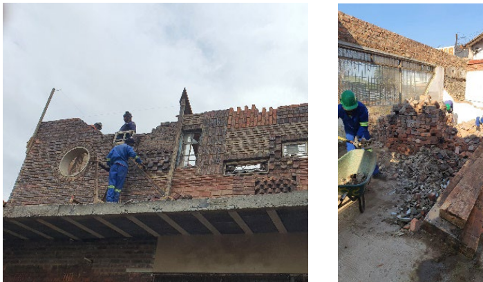
Figure 4.3 Proposed elevation showing reclaimed and salvaged brickwork. Photos of brick cleaning and bricklayer, Aaron Mahlangu, using creative licence to complete the façade (Author's drawing and photographs)
