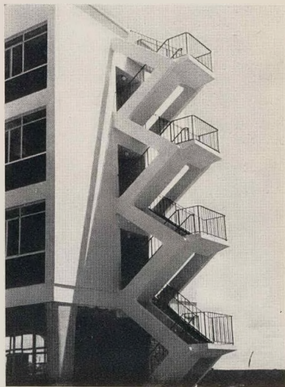
Below: The fire escape provides an accent of strong pattern at the end of each block, and is a tour-de-force of cantilever construction.
