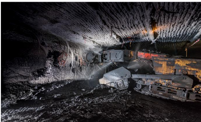
Figure 20 Drilling and blasting trucks
