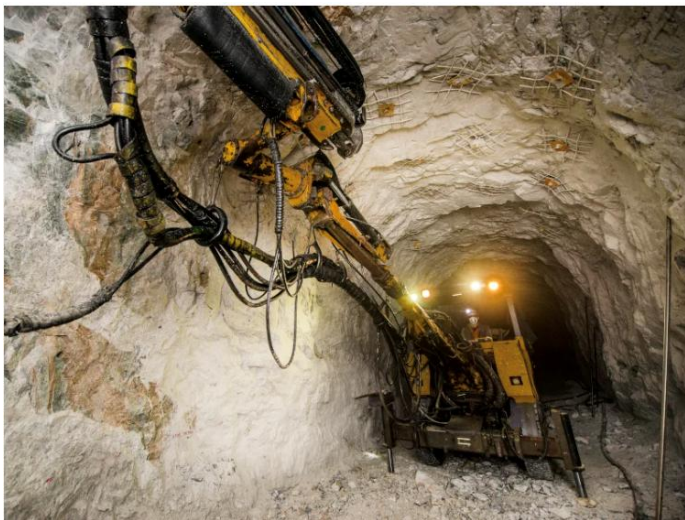
Figure 22 Tunnelling and exaction trucks
