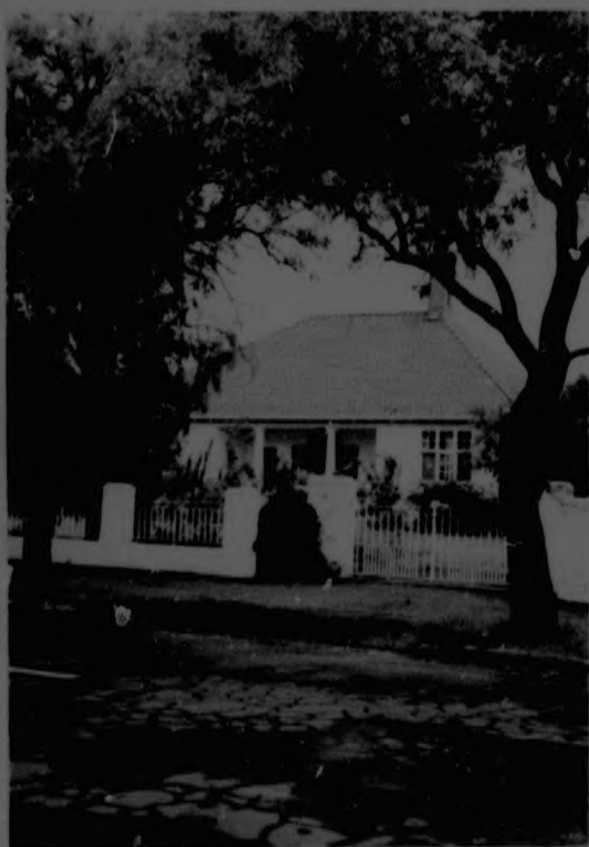
Baker's only known house in Kimberley dating to about 1905. It appears to have had no influence on subsequent houses of pre-1914 Kimberley.
