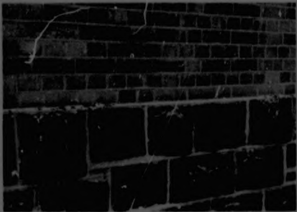
Dolomite foundation stonework under brickwork at Beit House. Built 1911.
