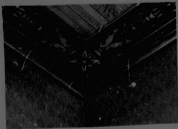
Belgrave Hotel foyer ceiling of wood grained matchboarding with stencil decorated surround on cloth.
