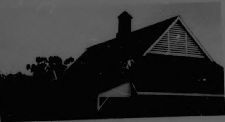
The ventilator on the ridge is connected by means of a duct to the classroom below. The louvre provides ventilation to the roof space. Kimberley Undenominational School.
