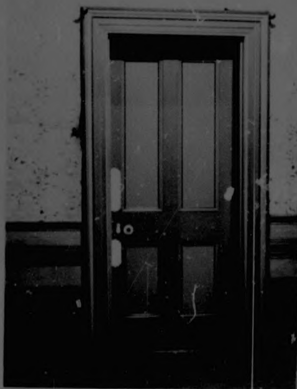
This single photograph taken in the entrance hall of The Bungalow (Rudd House) illustrates several of the excesses of late 1880's Kimberley decorating including door and architrave mouldings picked out in different colours, multi-coloured skirtings and striped cloth dadd.
