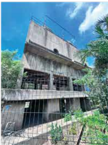
Figure 4.16 Existing Building on site
