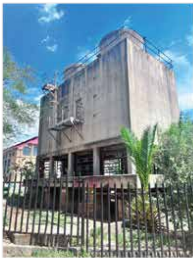
Figure 4.17 Existing Building on site
