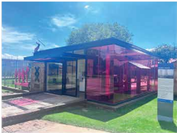
Figure 4.19 Workers Museum Entrance
