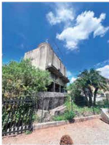
Figure 4.18 Existing Building on site
