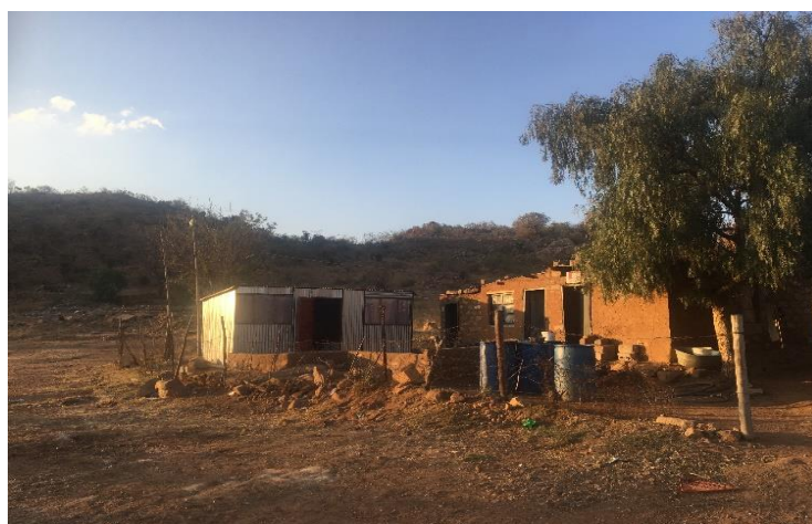
Plate 5: A tin shack built by the mine in replacement of a mud house that collapsed
