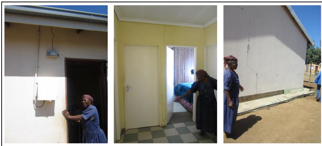
Plate 7: Cracks in a neighbouring house in Sterkwater village
