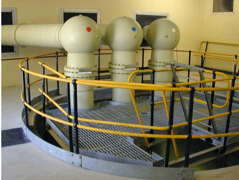
Figure 1.1: Surface exit of the Drakensberg Pump Storage station 400 kV GIS, used with permission
