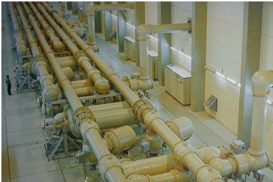
Figure 1.5: Alpha substation sited at 1500 m above sea level on the South African Highveld, used with permission
