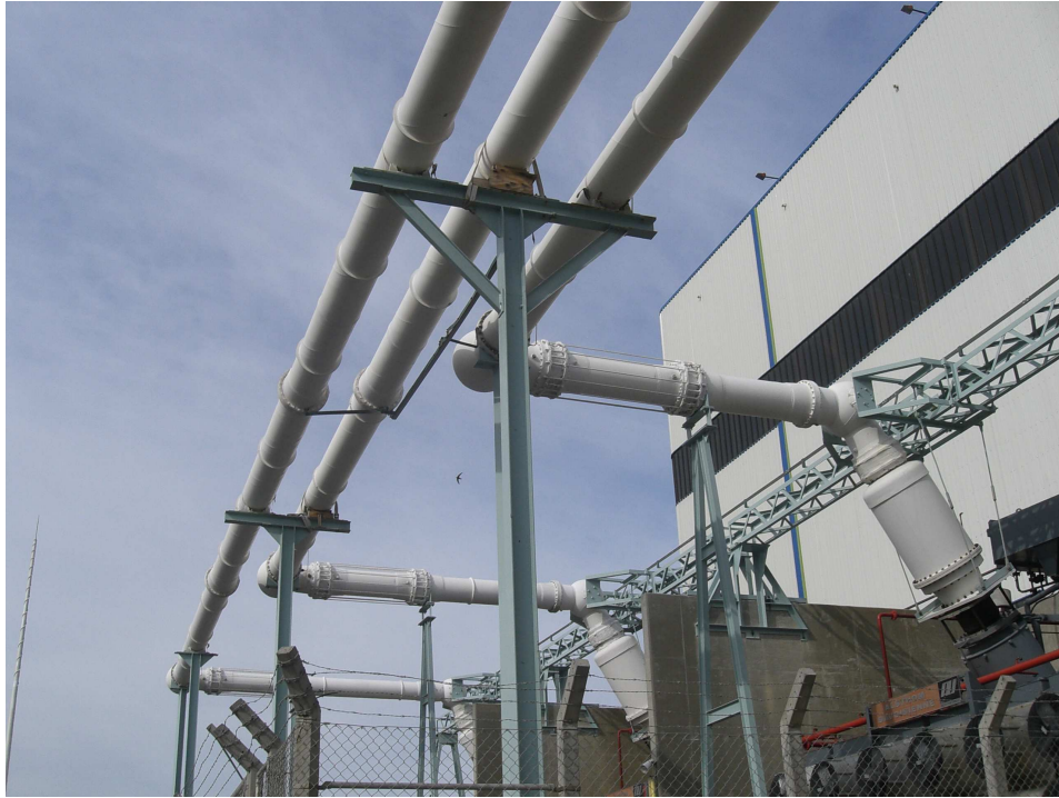
Figure 1.4: GIL installation at the Koeberg Nuclear Power Station en route to switch yard, used with permission
