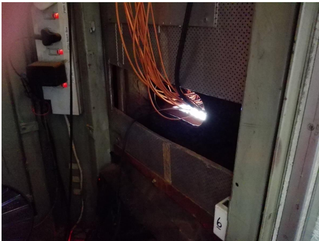
Figure 94: Photograph showing the fiber optic cables entering one of the Transnet Freight Rail test coaches.
