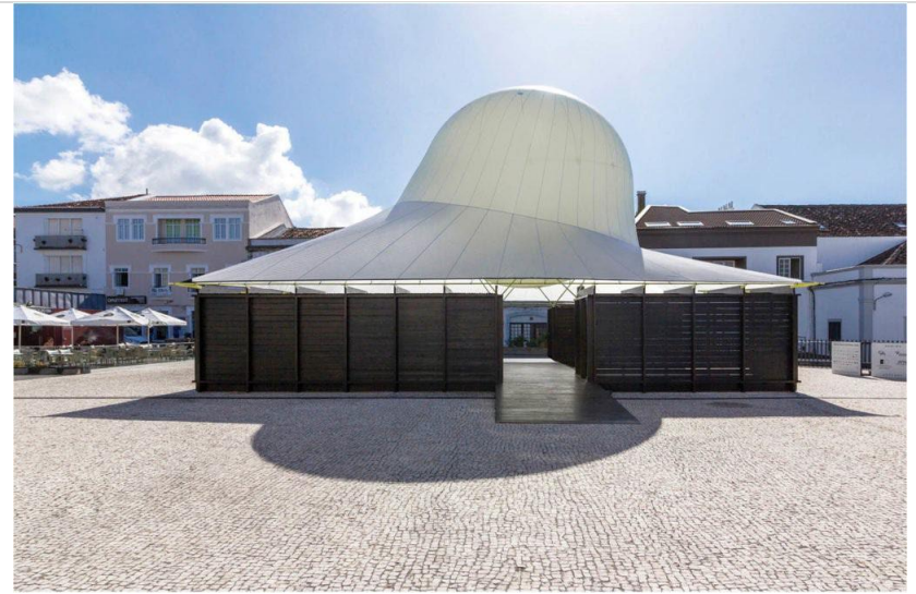
Figure 66: An example of dismountable structures , this temporary pavilion was designed by GA estudio + ArtWorks for the 2019 Festival de las Artes Walk&Talk event held in Portugal. The fabric roof, held up by an inflatable balloon, is anchored to movable modules housing exhibits.
