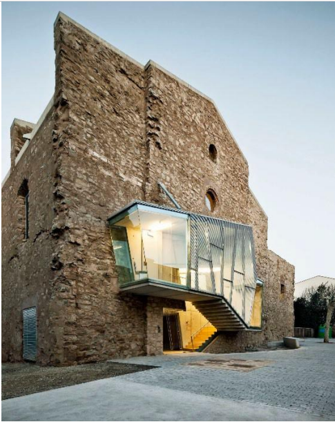
Figure 65: The convent of Sant Francesc church, which is located in Catalan, Santpedor was intended to be changed into a cultural facility. David Cross using symbiotic architecture in the form of parasitic architecture managed to allow the church to host a new auditorium and multipurpose center to be used as a cultural space. The upper floors were altered to become historical archives using existing roof volume space. This building well informs how to create a symbiosis between old and new.
