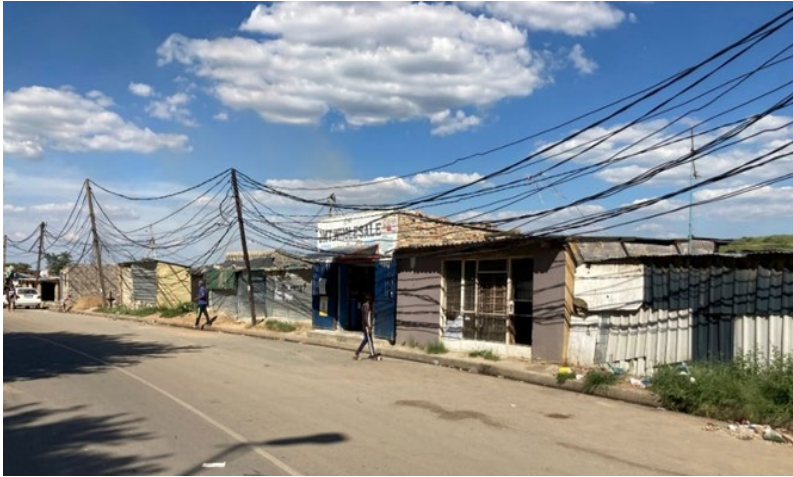
Figure 5.9 Illegal electricity connections by the community in Kya Sands (Source: Hopa, Kya Sands, 2022)
