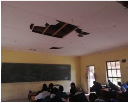
Image 1: Falling ceiling
