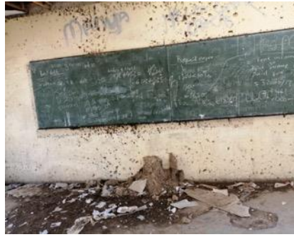
Image 2: Mould inside the classroom
