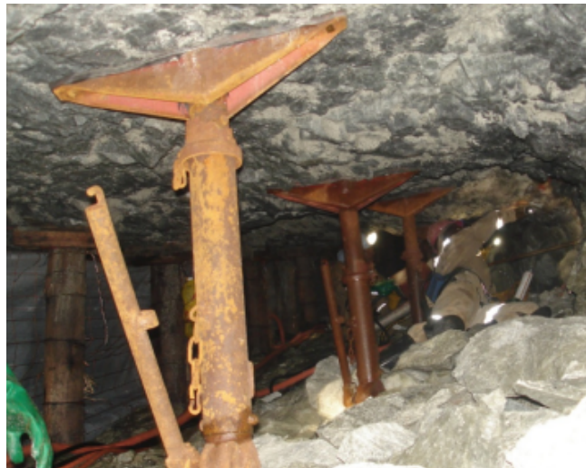
Figure 4.4: Temporary support made of mechanical props installed close to the face in a conventional mine (Ferreira 2012).
