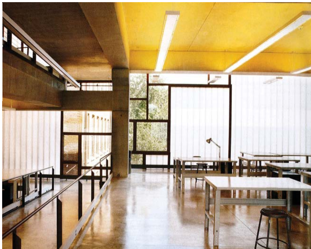
First floor showing the robust interior (four corner concrete columns and rusted steel handrails)
