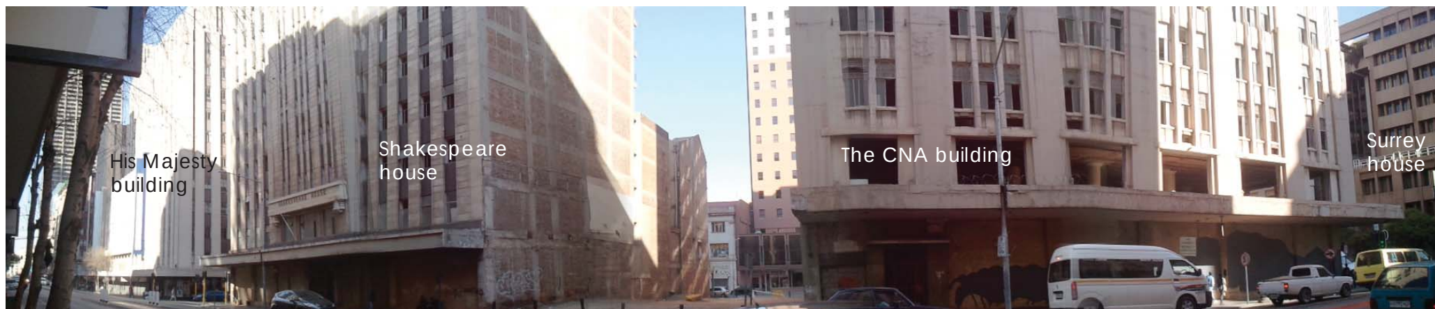
Shakespeare house and The CNA building Along commissioner street looking south, taken by: S.Mvumbi (2012)
