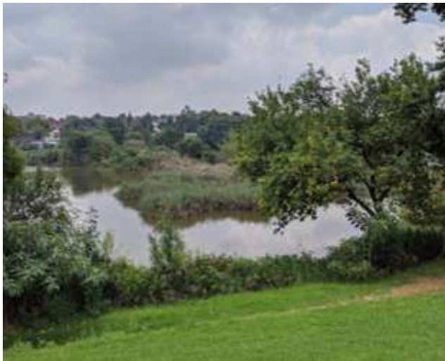
Edges around the dam
