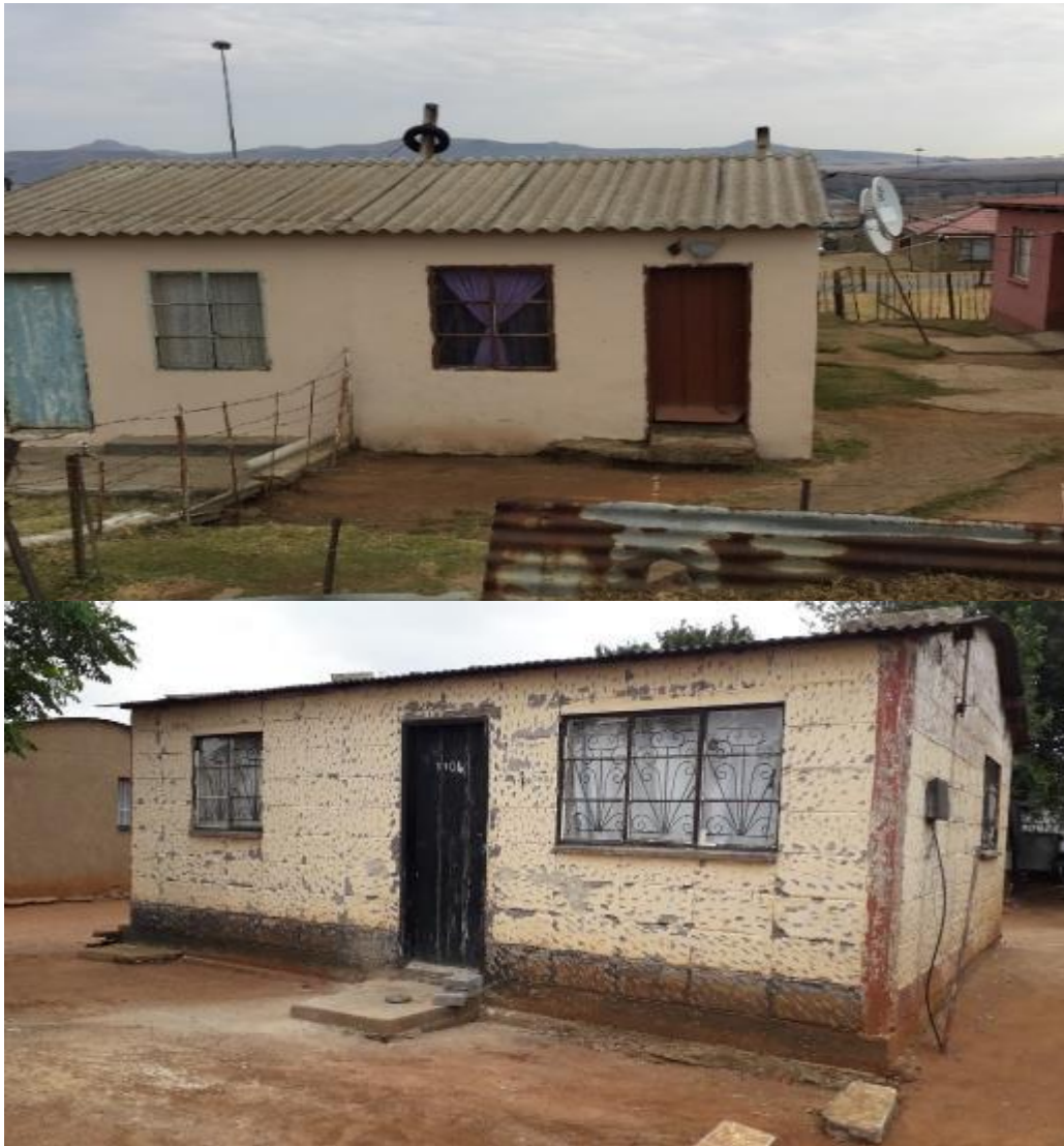
Figure 14: Two sub-types of apartheid era (matchbox) houses found in Wakkerstroom
