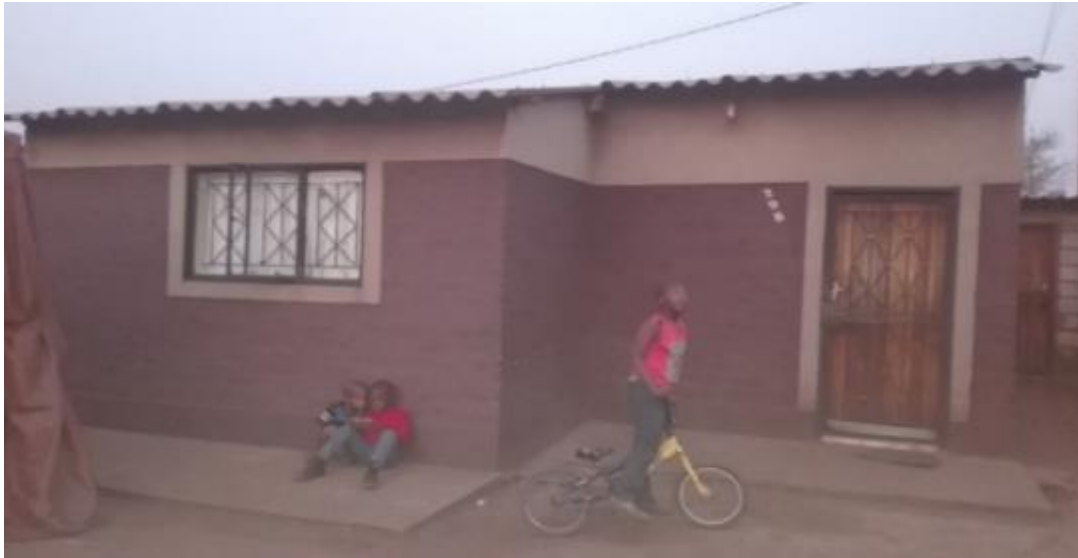
Figure 12: A distinctive RDP house in the Kathorus area, built in the mid- to- late 90s.
