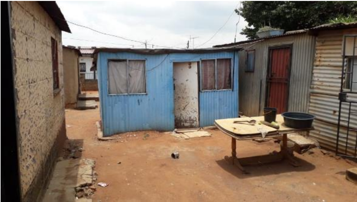
Figure 13: A typical backyard informal house (shack) in the Kathorus area.
