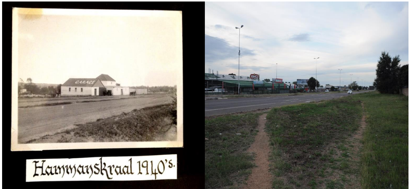
Figure 3: The earliest 16 picture of Hammanskraal against one in the year 2020 of the same point position.
