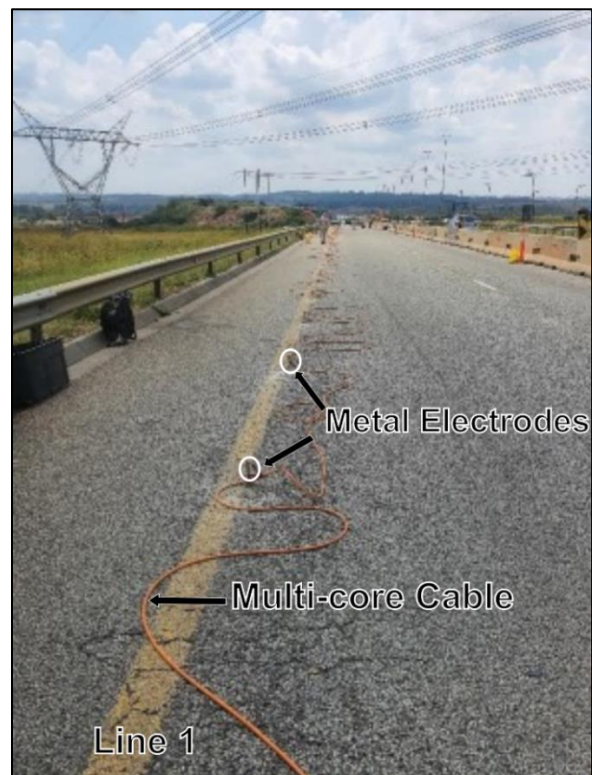
Figure 6.6: The profile of line 1 with metal electrodes of a 2.5 m spacing on the R21 tarred surface.
