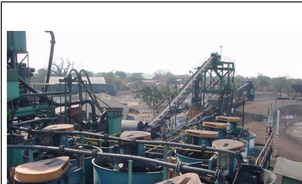
Figure 1.7: Wemco Flotation cells installed in 1996
