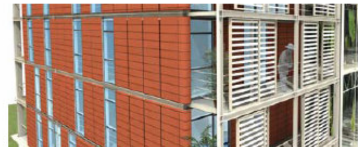
SW Balcony view
