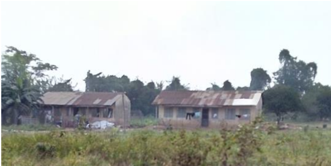
Fig.5.19 Old residential buildings of Farm Settlers, Akufo Farm Settlement, Akufo, Ido LGA (Source: Author, 2020)
