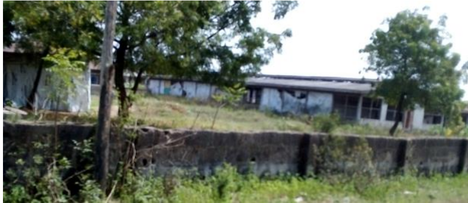
Fig.6.3 The only functional Pen at the extreme corner of the moribund Ejioku Farm Project (Source: Author, 2020)
