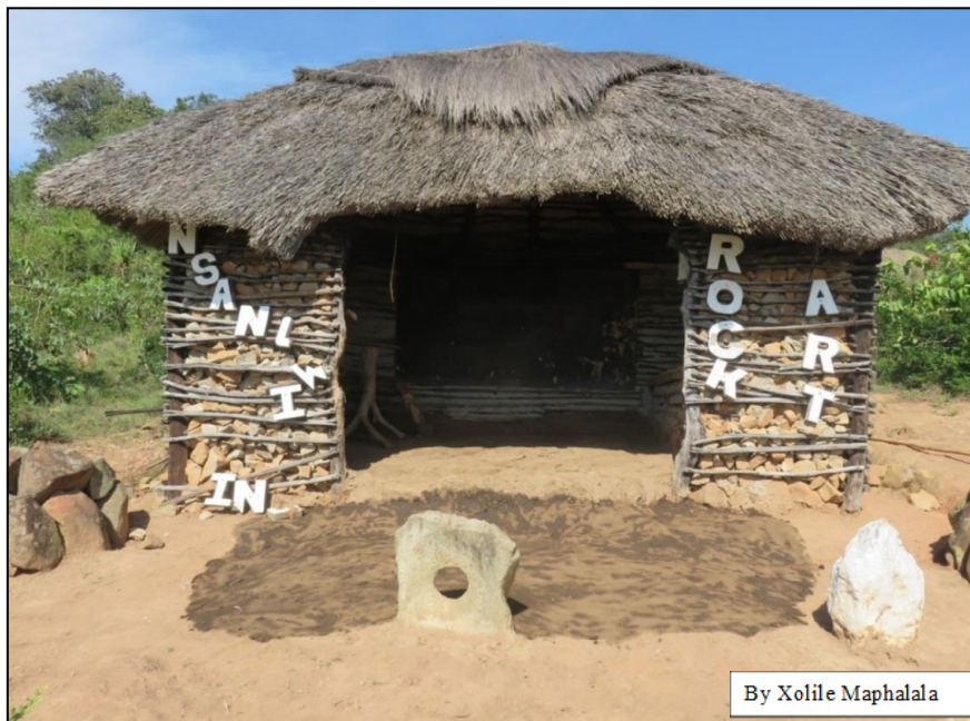
Figure 7: Reception to Nsangwini rock art experience, built using local materials and traditional methods. Note the fresh dung floor and grindstone.
