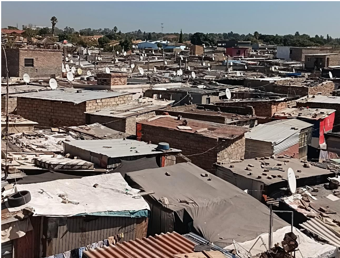
Figure 6: Image showing density and building materials e.g. corrugated iron sheets, fabric, bricks (Source: Author, 2024)
