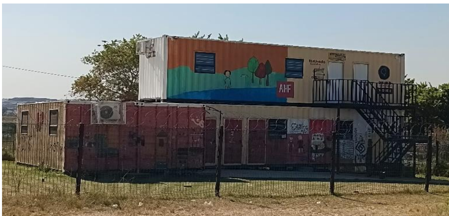
Figure 15: Nthethelelo Foundation, made from shipping containers and fenced for security and limiting access. Source (Author, 2024)
