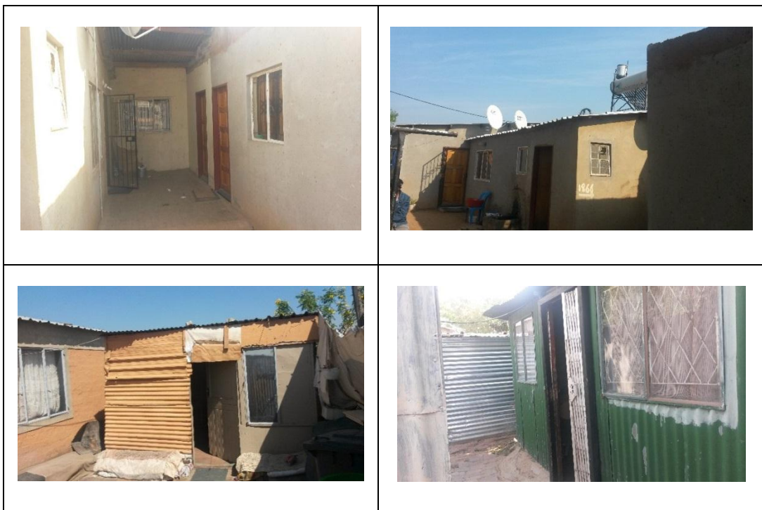
Figure 15: (Clockwise left to right), Multiple backyard dwellings neatly constructed, arranged for maximum income in Cosmo City vs. the corrugated backyard shacks found in Diepsloot (Source: Kevin Chetty)
