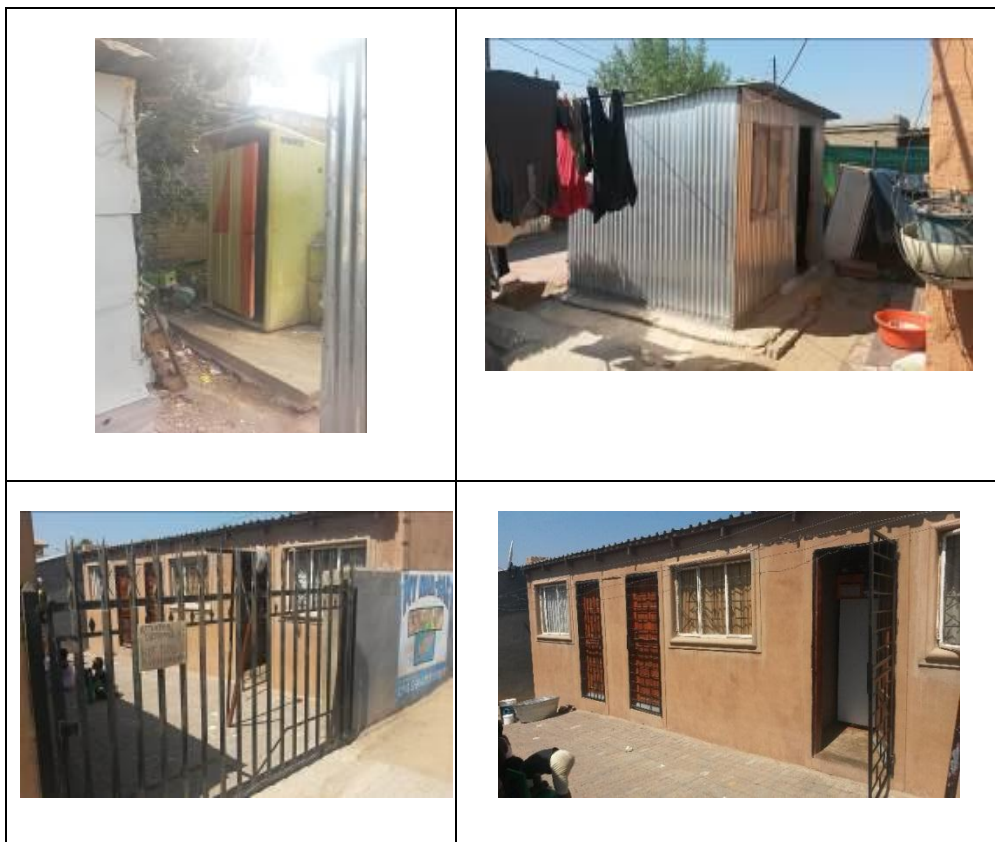
Figure 17: (Diepsloot, Clockwise left to right), Services informally provided includes central ablution facilities, electricity informally and illegally connected from main house, well-structured units with front gates, and added security (Source: Kevin Chetty)
