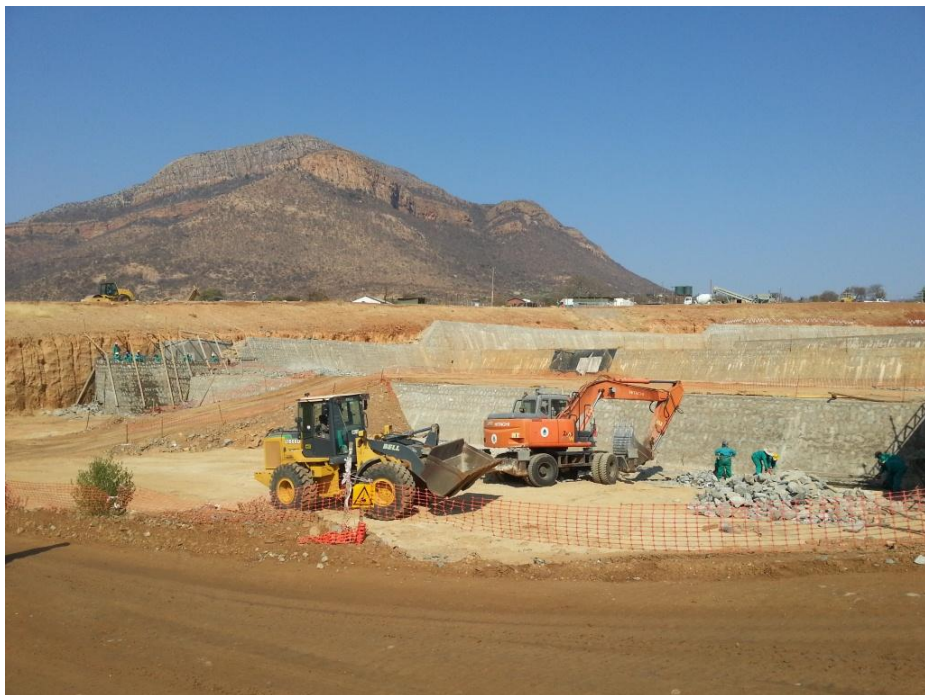
Figure 3.9: Chuniespoort Dam spillway construction (2)
