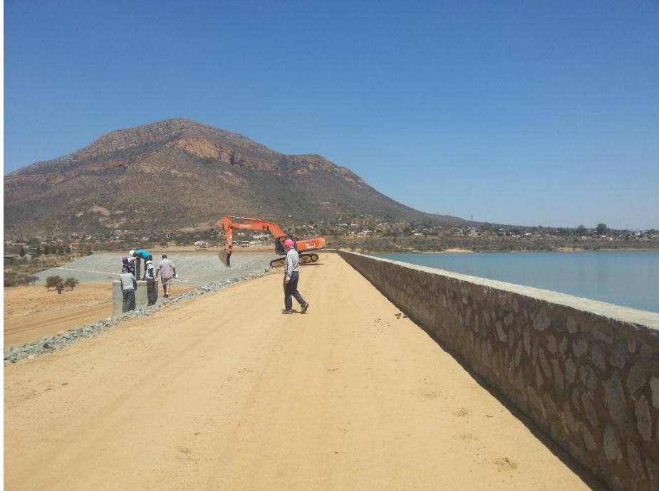
Figure 3.10: Chuniespoort Dam parapet wall
