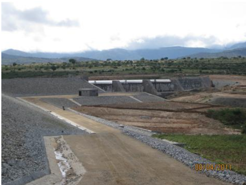
Figure 3.6: Molepo Dam completed
