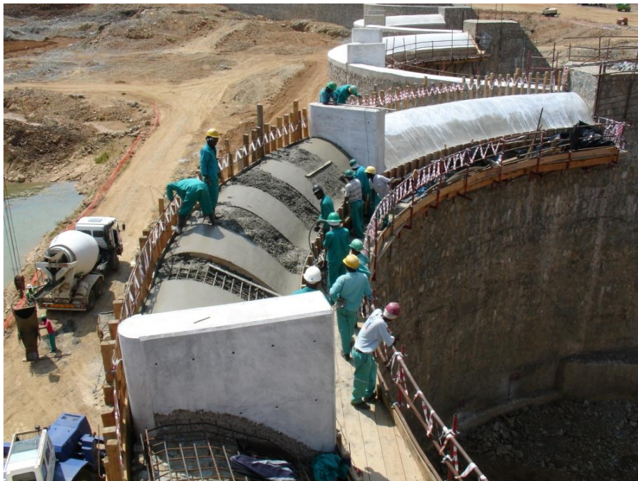
Figure 3.4: Molepo Dam spillway ogee profile during construction
