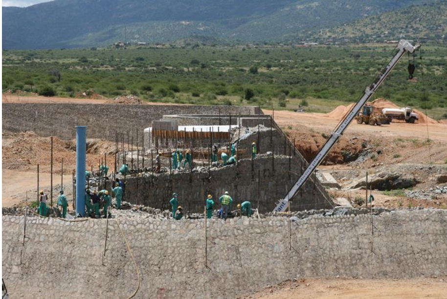
Figure 3.3: Molepo Dam spillway during construction (3)
