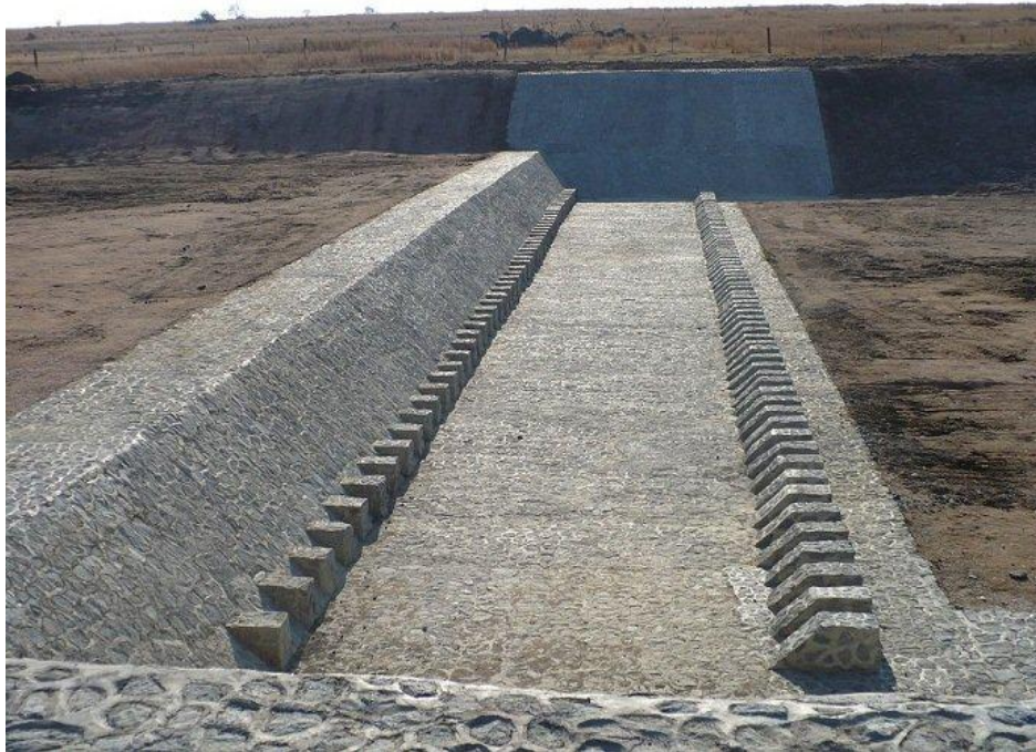
Figure 3.16: Mashashane Dam completed spillway
