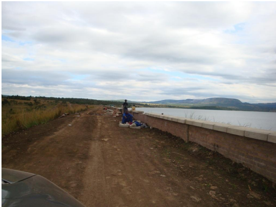
Figure 3.20: Albert Falls Dam during construction of the parapet wall
