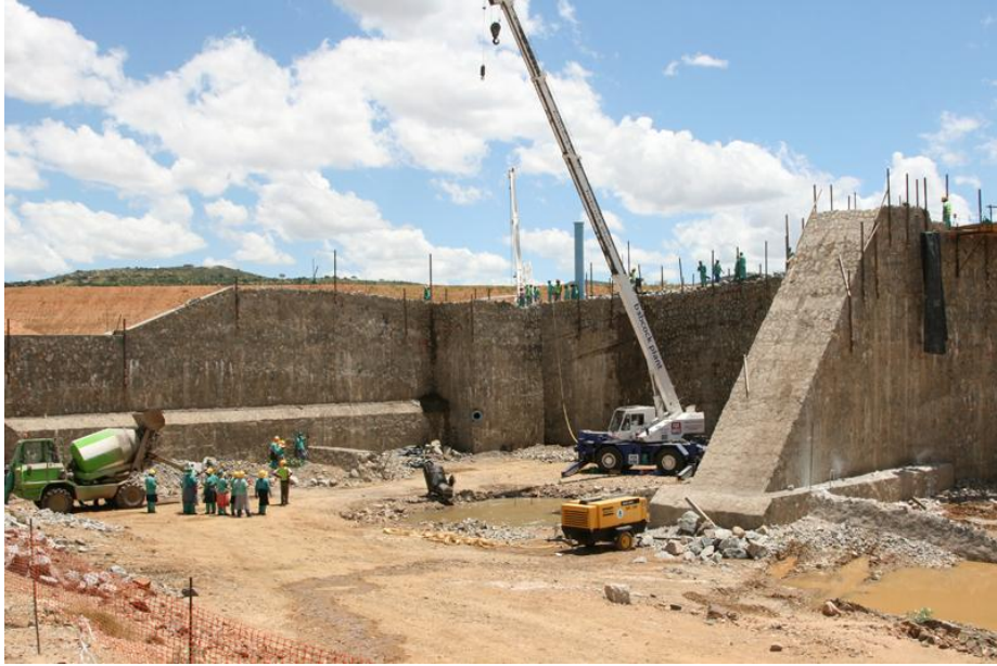
Figure 3.1: Molepo Dam spillway during construction (1)
