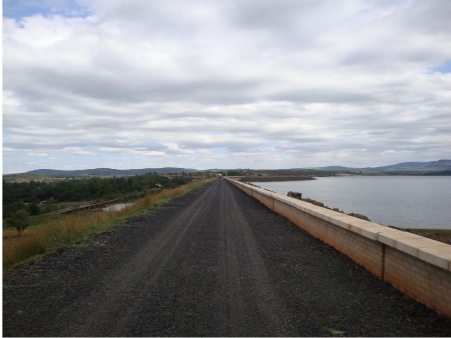
Figure 3.21: Albert Falls Dam completed parapet wall
