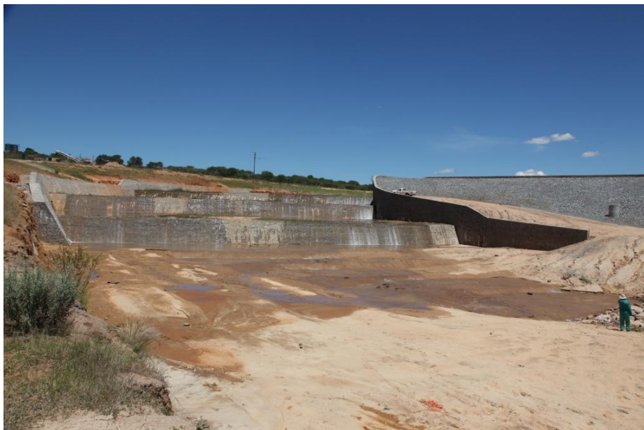
Figure 3.13: Chuniespoort Dam completed rubble masonry concrete spillway
