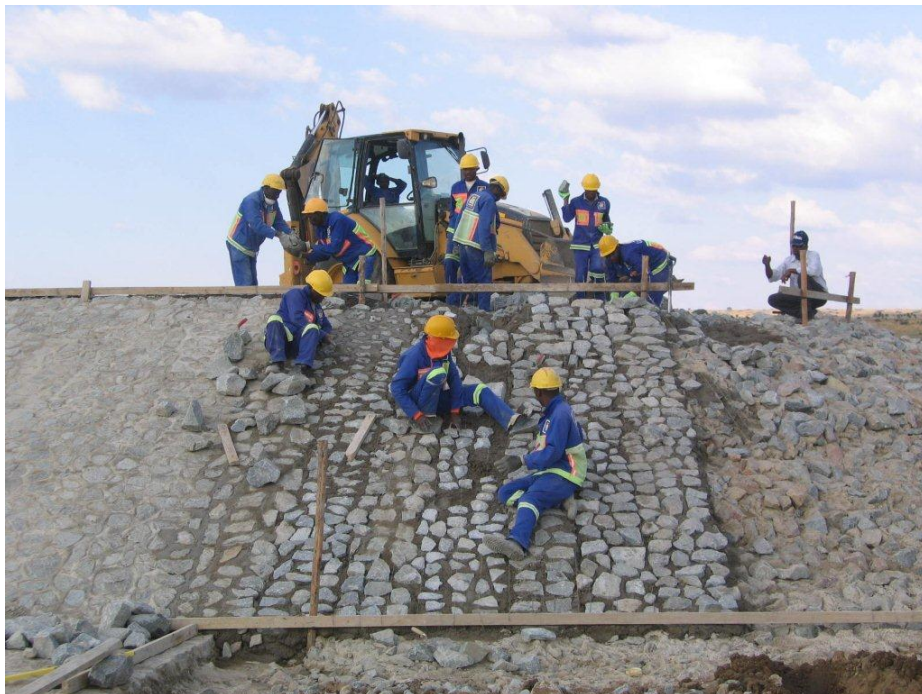
Figure 3.15: Mashashane Dam spillway during construction (2)
