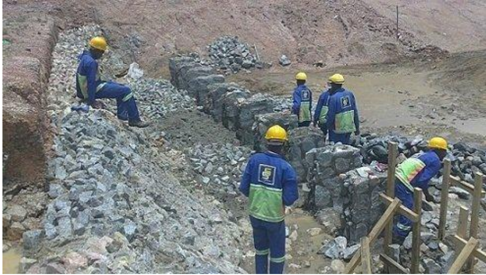
Figure 3.14: Mashashane Dam spillway during construction (1)
