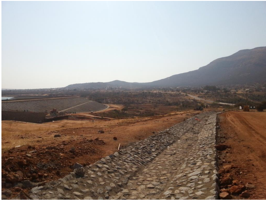
Figure 3.12: Chuniespoort Dam stormwater canal
