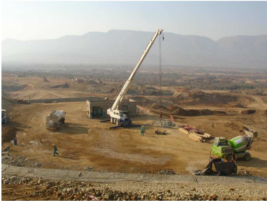
Figure 3.5: Molepo rubble masonry concrete pump house during construction
