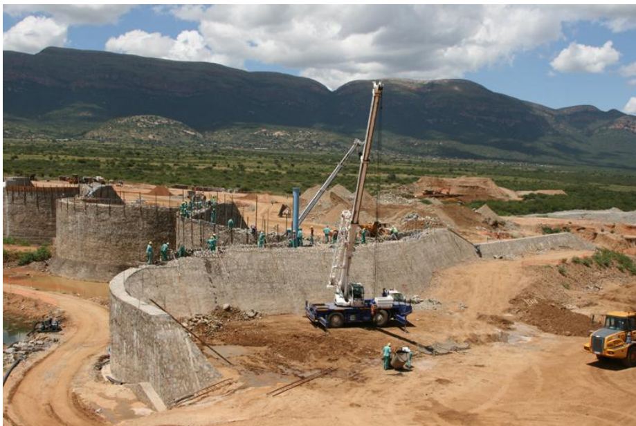
Figure 3.2: Molepo Dam spillway during construction (2)
