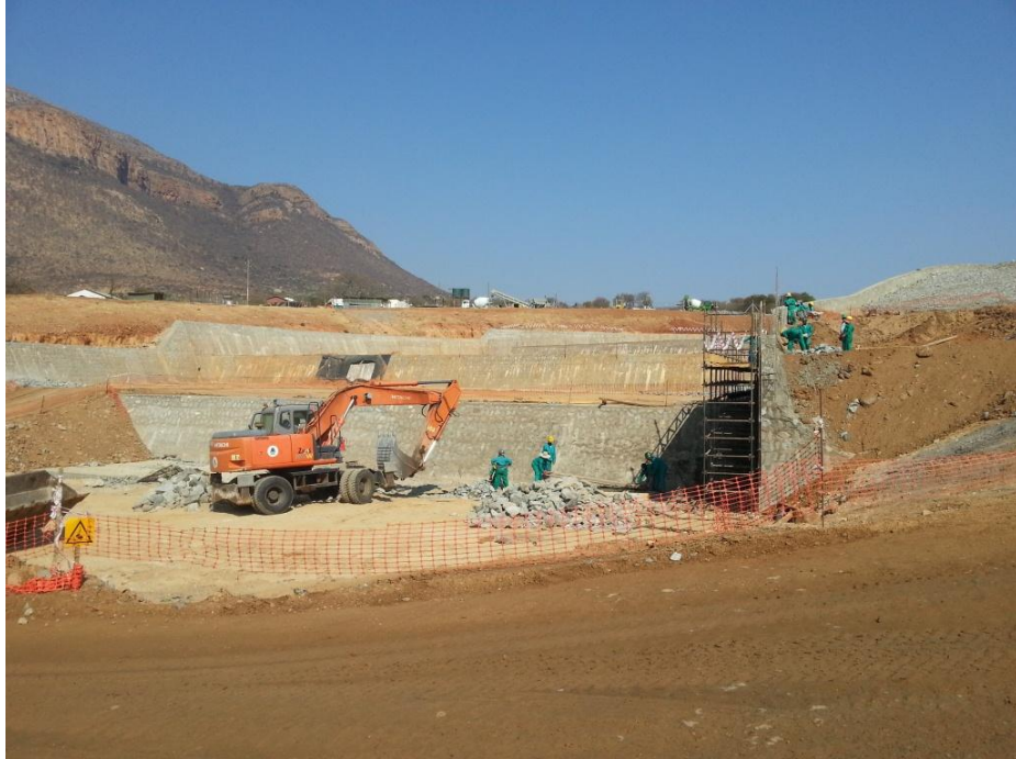
Figure 3.8: Chuniespoort Dam spillway construction (1)
