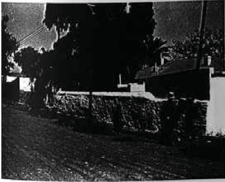
Erf 588: Back wall of 66 Church Street.
