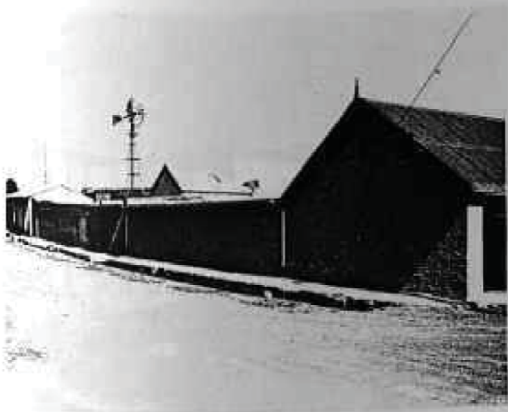
Erf 506: Back wall of 84 Church Street.
