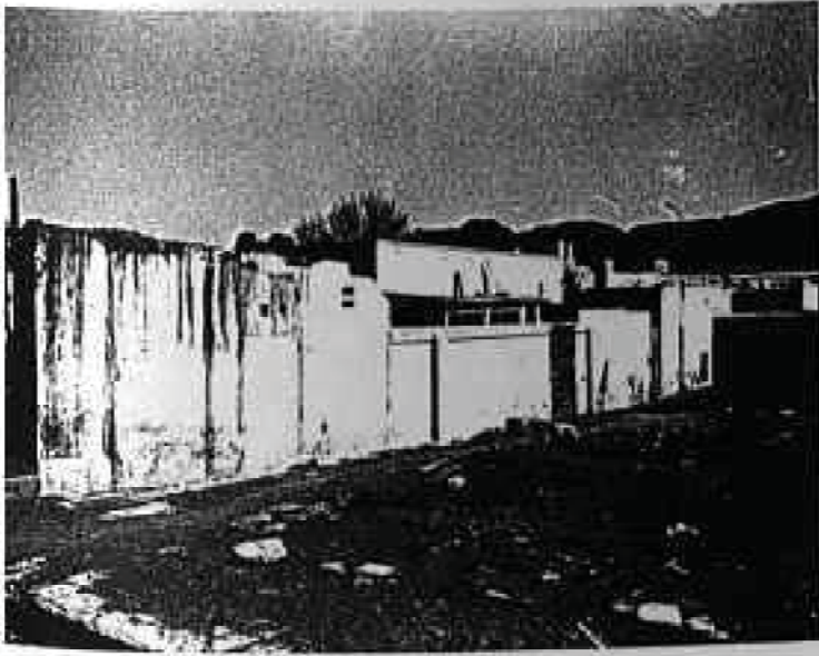
Erf 523: Remains of alley wall, Campbell Street.
