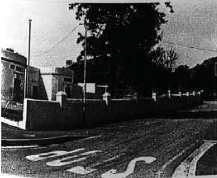
ref 1168: ? New Street (prev. Mimosa House).
