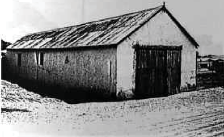
Erf 533: Shed, Campbell Street.
