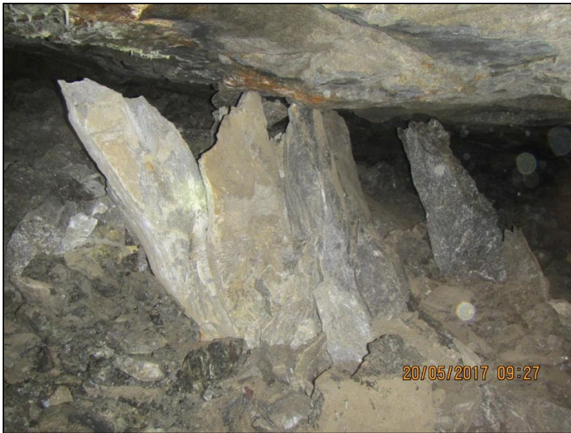
Figure 13: Rotation of footwall slabs due to footwall heave at 11-32W Merensky Reef panel
