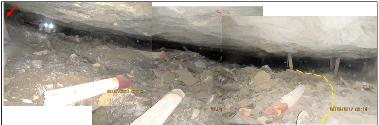
Figure 32: The footwall heave zone (approximately 10 m radius) around the failed Merensky Reef pillar. The red arrow indicates the pillar position
