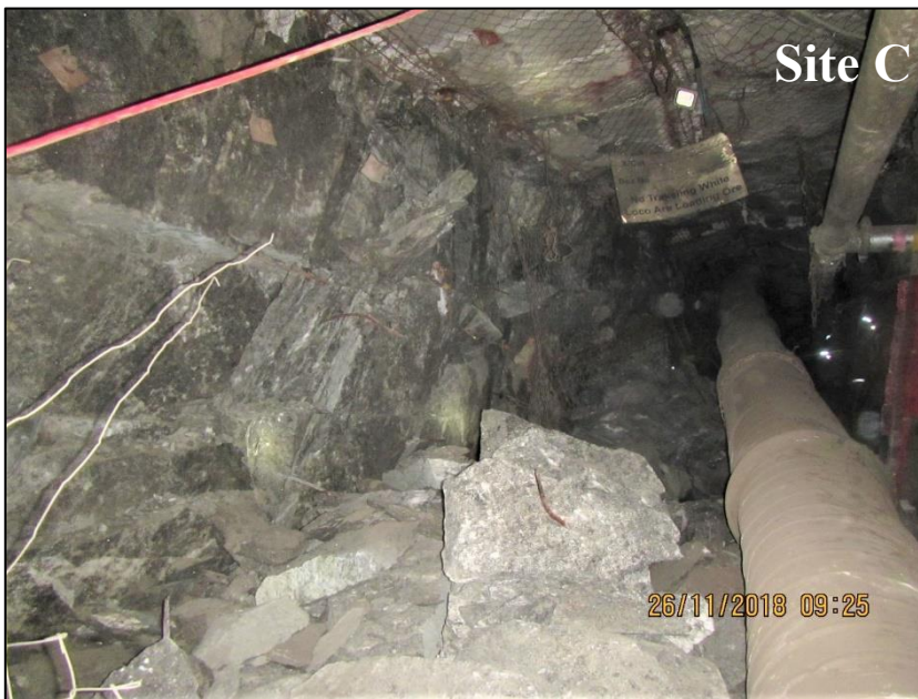
Figure 75: 14-23W UG2 crosscut - western sidewall
