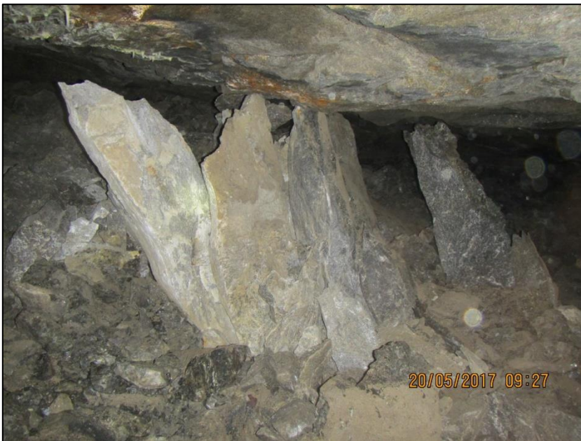
Figure 34: Rotation of footwall slabs due to footwall heave
