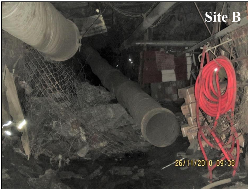
Figure 74: 14-23W UG2 crosscut at the entrance to the travelling way to the raise - western sidewall
