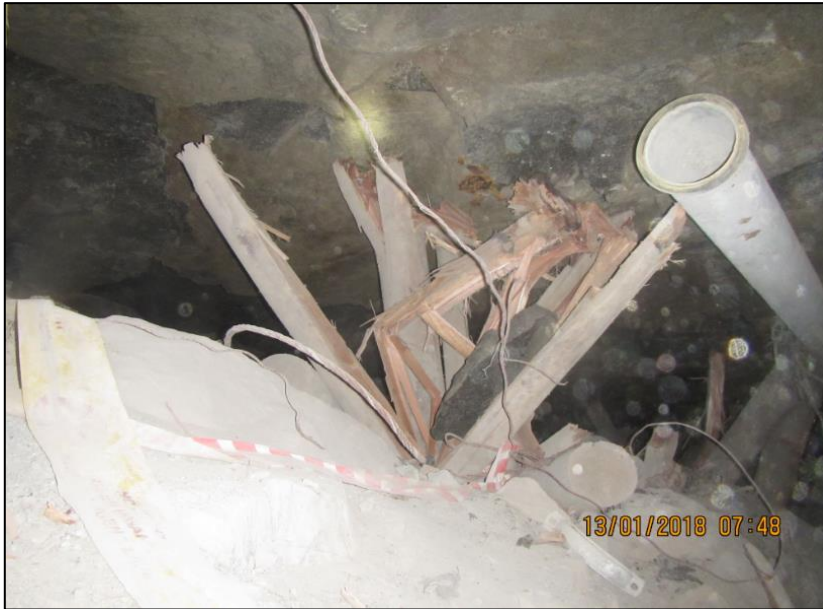
Figure 48: Very high closure of the Merensky Reef panels. Photo taken in the centre gully
