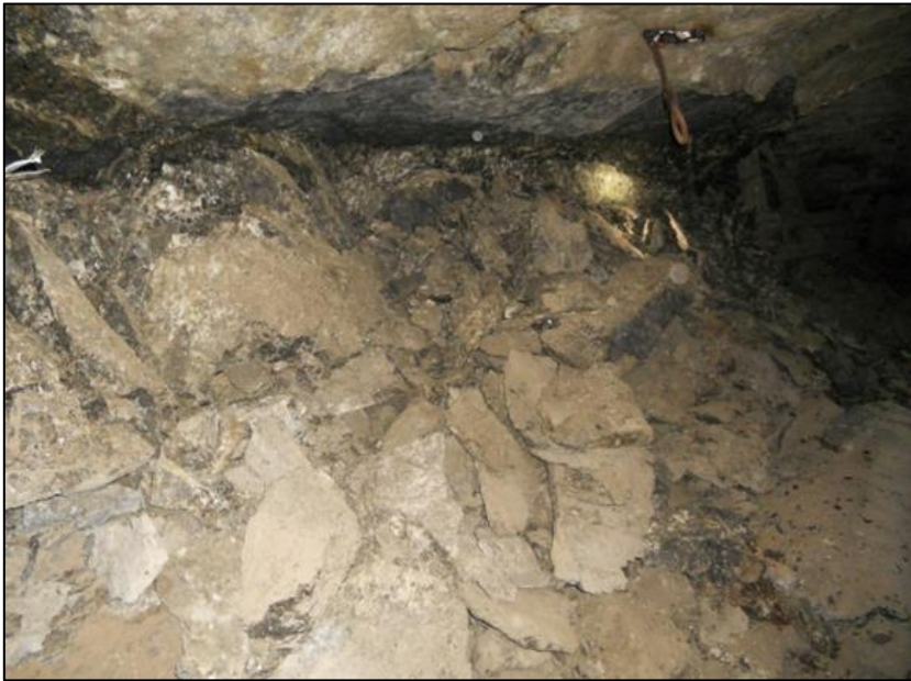
Figure 40: The failed Merensky Reef pillar
