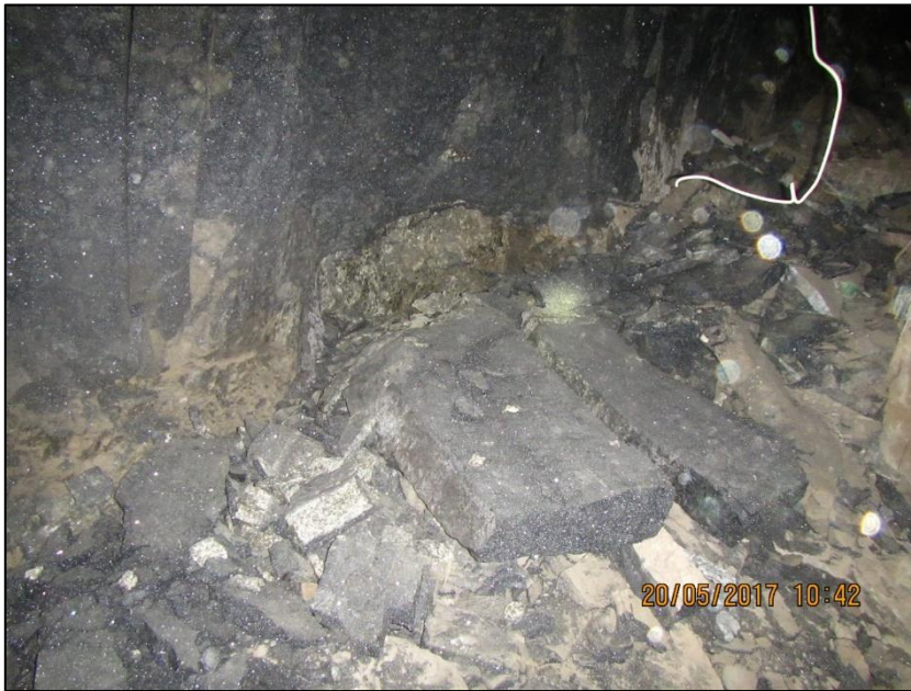
Figure 35: The superimposed UG2 Reef pillar, which had little sign of damage
