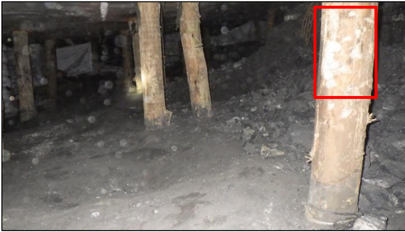
Figure 82: The 14-20W 4E panel showing pillar remnants in the panel and the marks on the timber elongates
