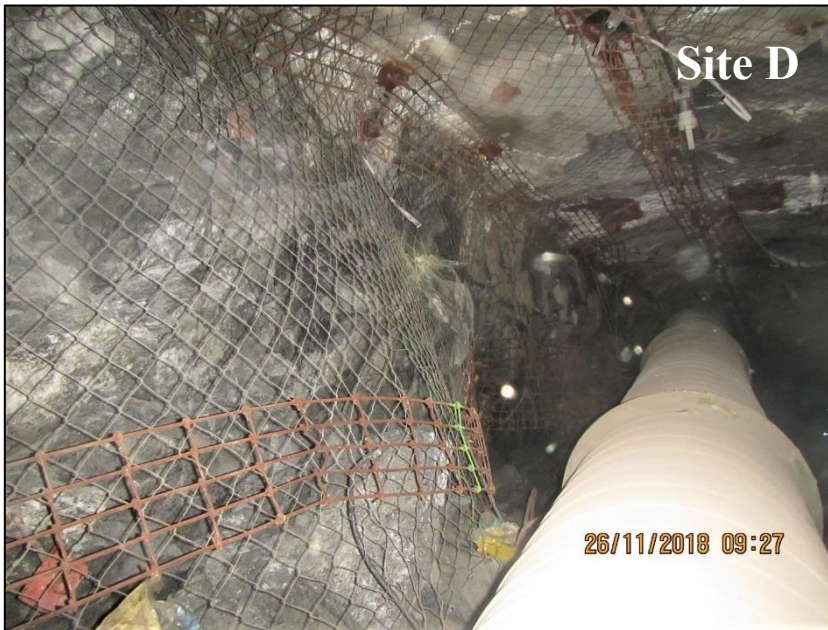
Figure 76: 14-23W UG2 crosscut - western sidewall
