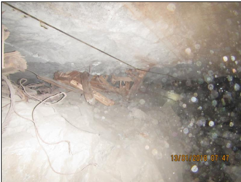
Figure 47: High closure of the Merensky Reef panels. Photo taken in the centre gully
