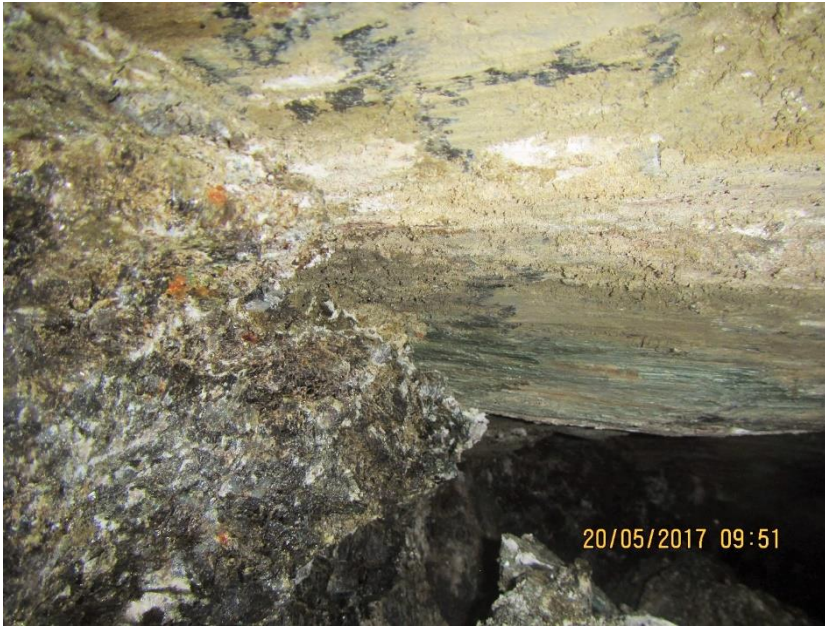
Figure 30: The failed Merensky Reef pillar. Movement along a contact plane between the pillar and the hangingwall
