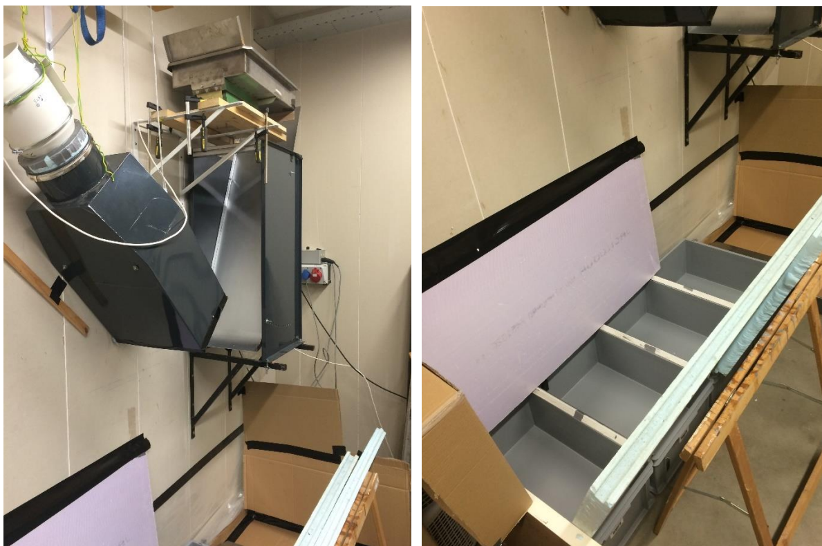
Ballistic separator with air knife in place
