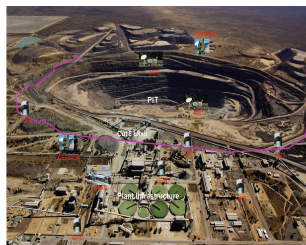
Figure 6—Monitoring equipment positioning
