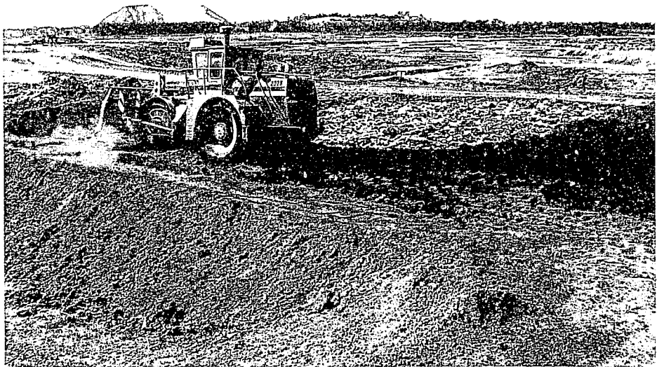
Plate 7.7 Compaction and covering of refuse
