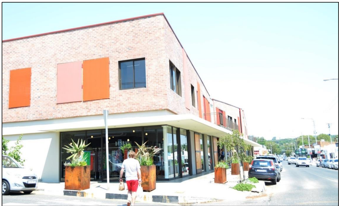
Figure 18 More Recent Development on 4th Avenue (Kok, 2015)
