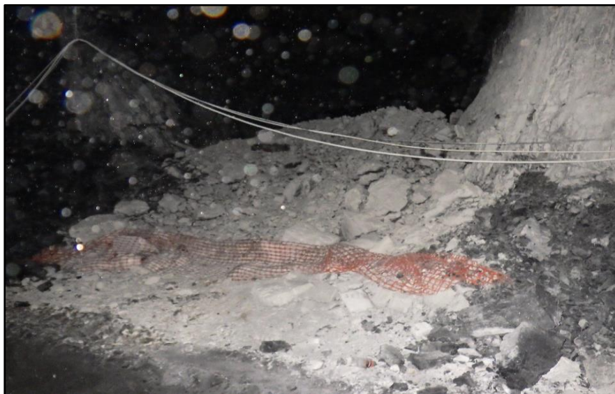
Figure 3.2-1- Hourglass shaped pillar formed by scaling at the No.2 Seam in Goedehoop colliery ( AngloAmerican (Thermal coal), 2017 )
