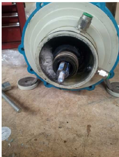
Figure 25: KOH crystal formation at high concentration and temperature resulting in rapid degradation of the chemical pump mechanical seal.
