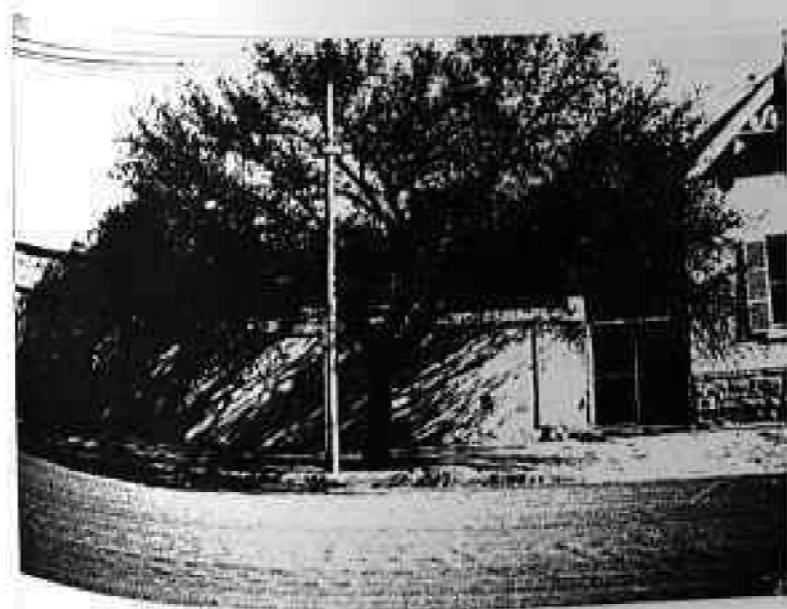
55/58. Erven 768/449: Wall between 3 & 5 d'Urban Row.
