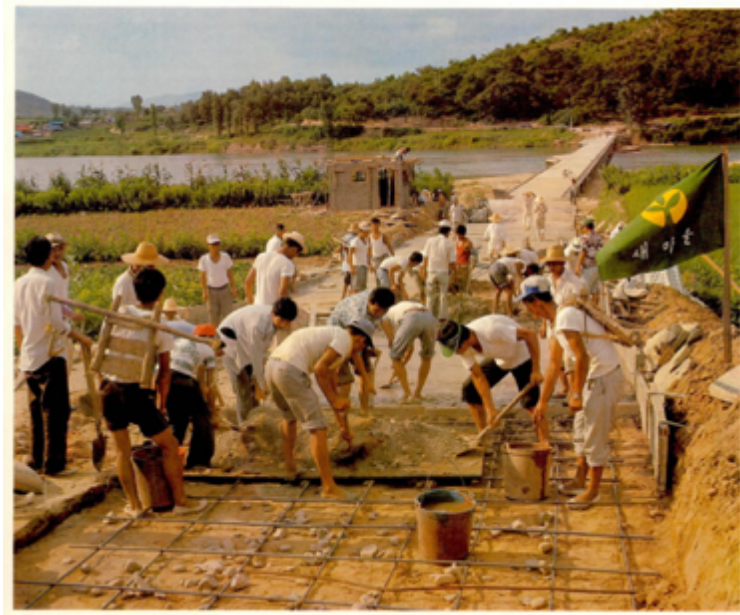
FIGURE 22. Villagers constructing a bridge for themselves according to the guidance of their Saemaul leader. Saemaul Pictorial (1979: 23). 64
