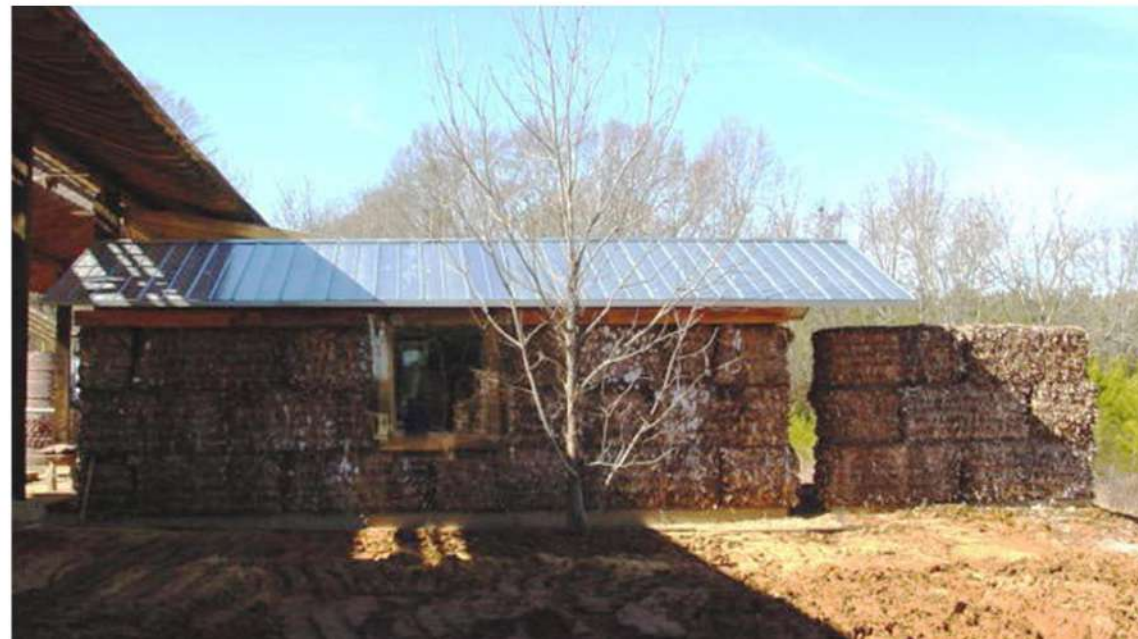
Fig 12 (a-f): Images of a corrugated carbon pod- an example of a building made using non-conventional building materials Rural Studio. 2001. Corrugated Cardboard Pod.
