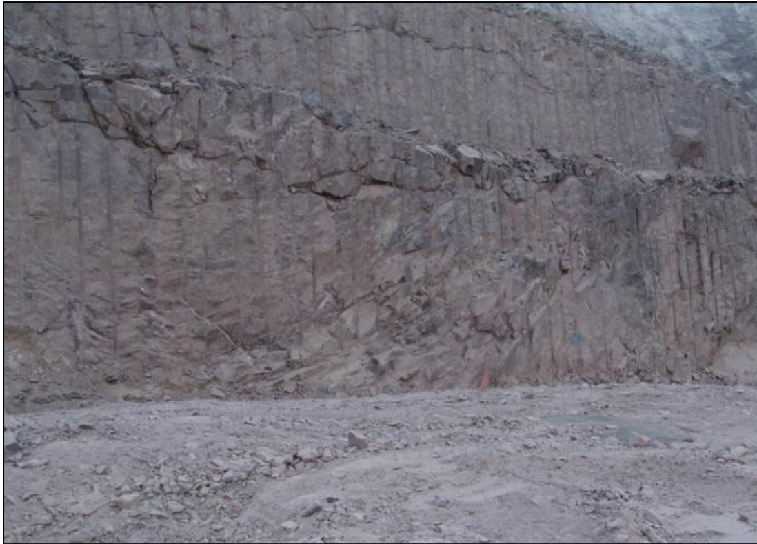
Figure 7.3 Photograph of a well pre-splitted and cleaned final limit bench in Structural Volume 1. Note the damage near the crest of the bench.
