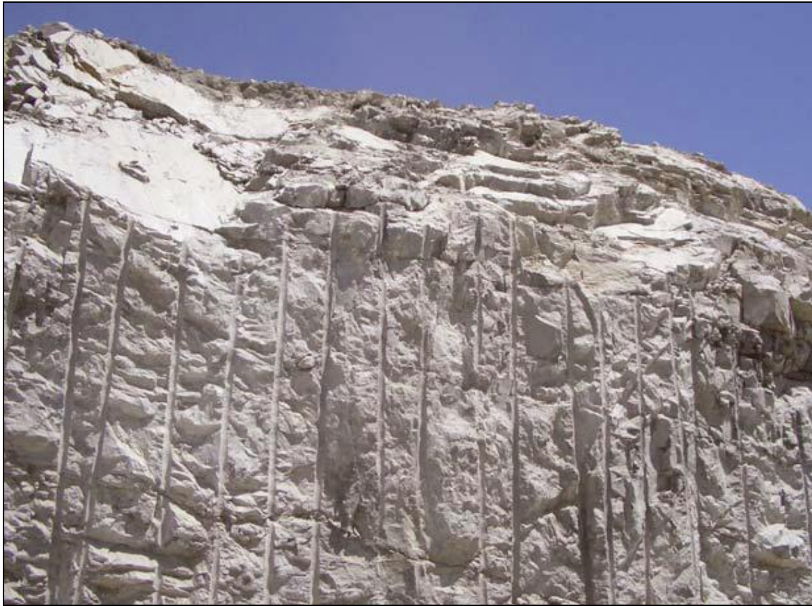
Figure 7.1 Photograph looking at the south wall, showing recent presplit results. The quality of the wall is very good, but the crest integrity could not be maintained.
