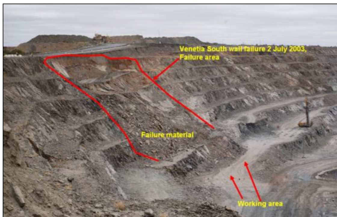
Figure 6.5 The largest failure to date in the Venetia pit (Tsheko, 2010) on 2 July 2003 in Cut 3.
