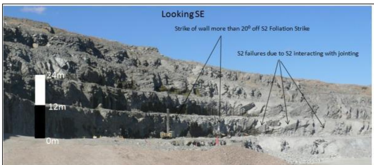
Figure 1.10 Photograph looking SE in the pit showing the S2 foliation in relation to the East Wall. Note how the planar failures decrease as the difference in strike between the S2 foliation and East wall increase.
