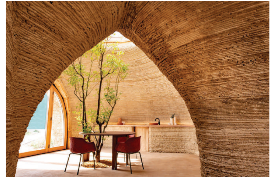
Figure 82 - Internal Photograph of TECLA 3D Printed Prototype (Mario Cucinella Architects, 2021)
