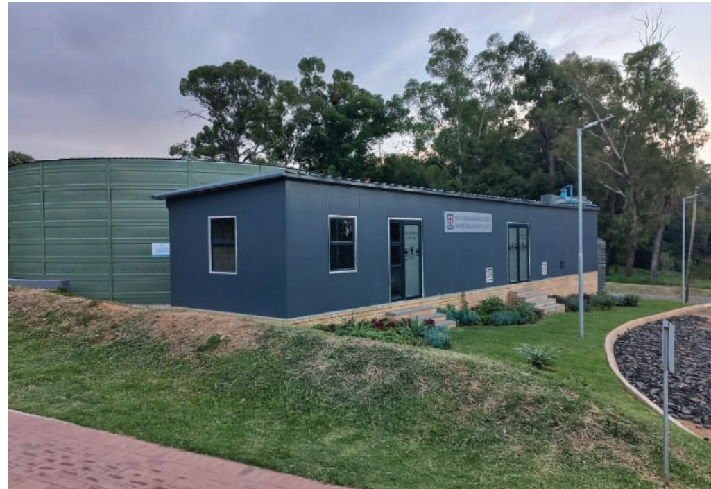
Figure 4 - St Stithians Water Treatment Centre – 07/05/2023
