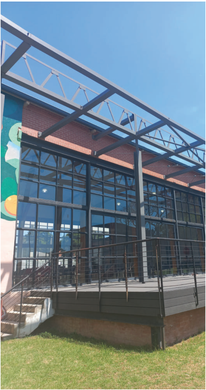
4. Hall with Kitchen and Deck
