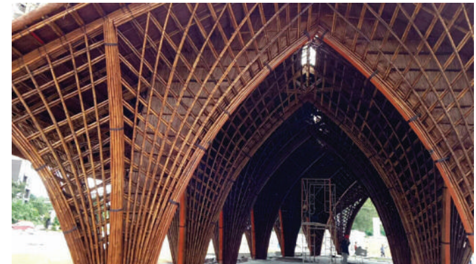
Figure 36 - Construction of Ting Xi Bamboo Restaurant
