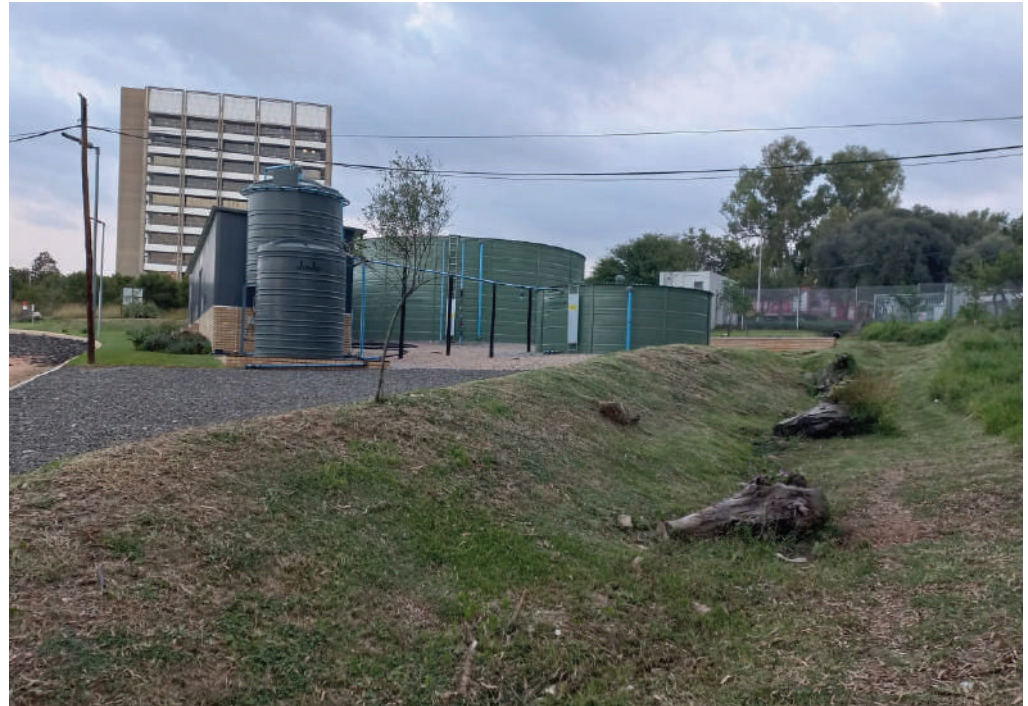
Figure 5 - St Stithians Water storage – 07/05/2023
