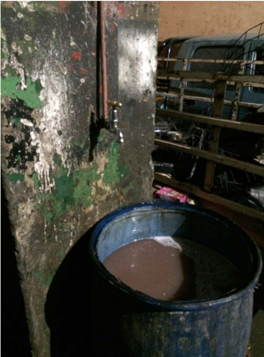
FIGURE 14: The only water source at the basement level, drainage is not a possibility without water pumps to ground level.
