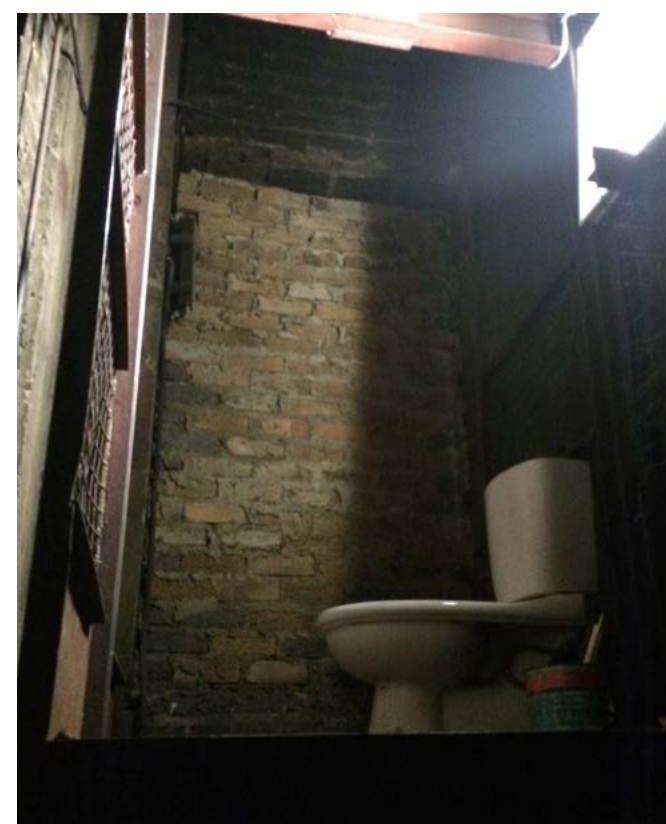
FIGURE 12: Toilet built in the old lift well
