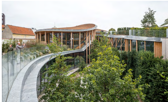
Image 23. (Hjortshøj, 2023) Looking from balcony to central courtyard
