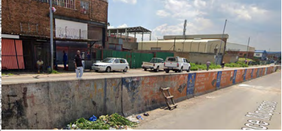
Image 37. (Google Maps, 2023) The barrier along Florence Moposo street is an inaccessible concrete wall which prevents pedestrians from crossing.
