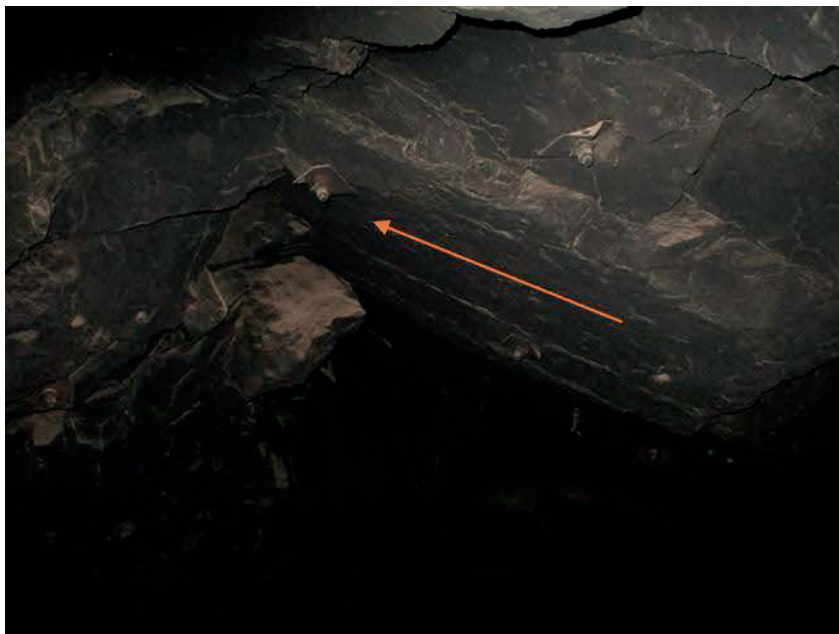
Figure 6.2: Flat dipping joint on hanging wall
