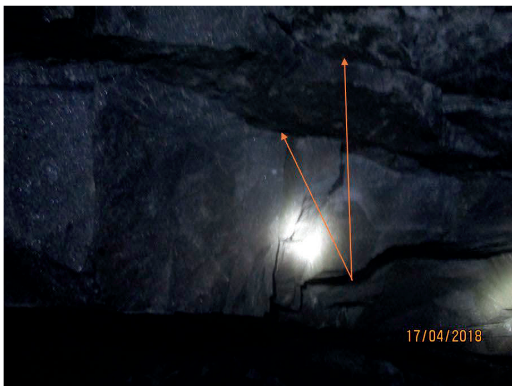
Figure 6.3: Horizontal parting planes in the hanging wall forming brows
