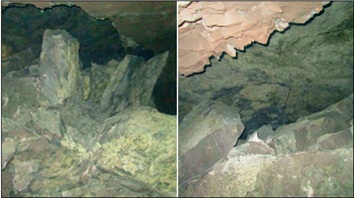
Figure 2.7: Fall of ground as a result of multiple parting planes with sepiertinite infilling ( Internal Mine Document, 2011 )
